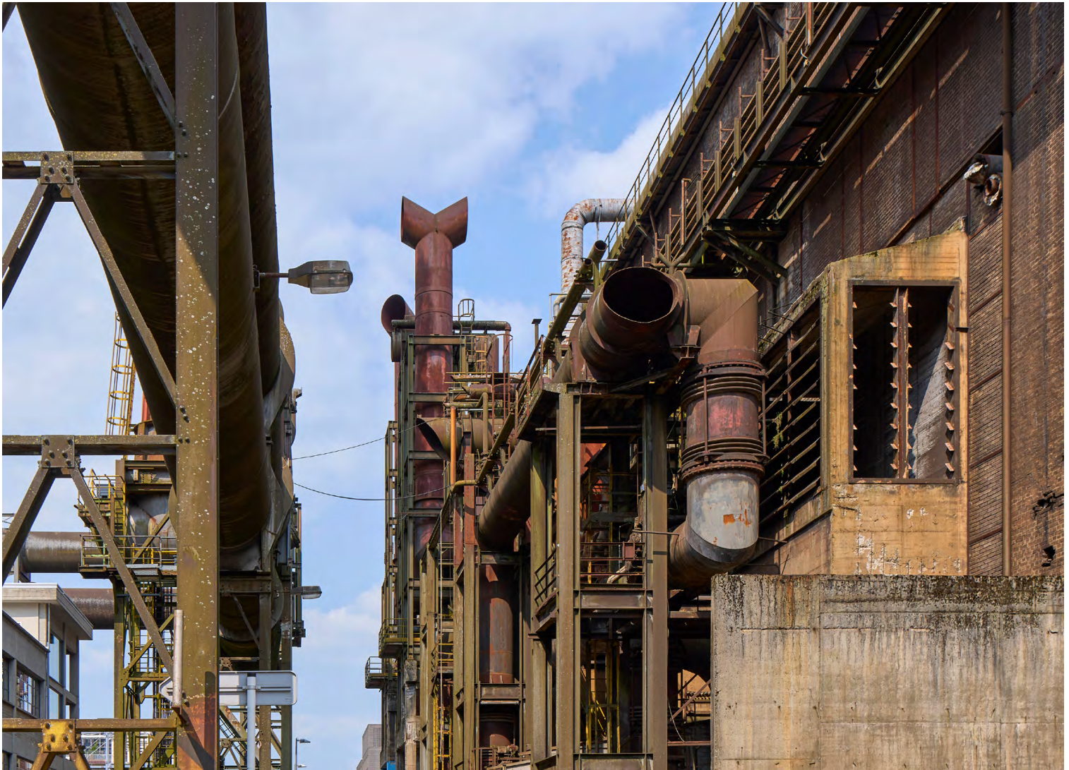
Blower hall at Esch-sur-Alzette, Luxembourg (photo by Eric Chenal, CC BY-NC-SA 4.0)
