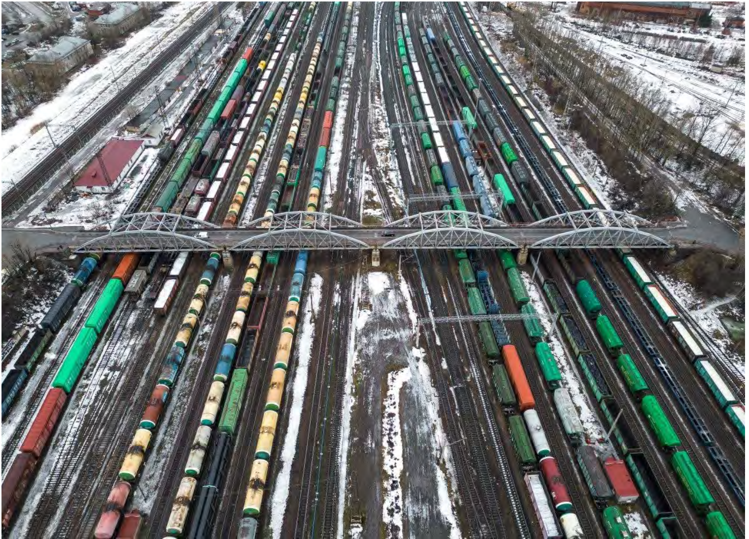
Farforovsky Bridge (Tsymbalinsky Overpass), drone footage, 2025 (photo by Oleg Mukhin)
