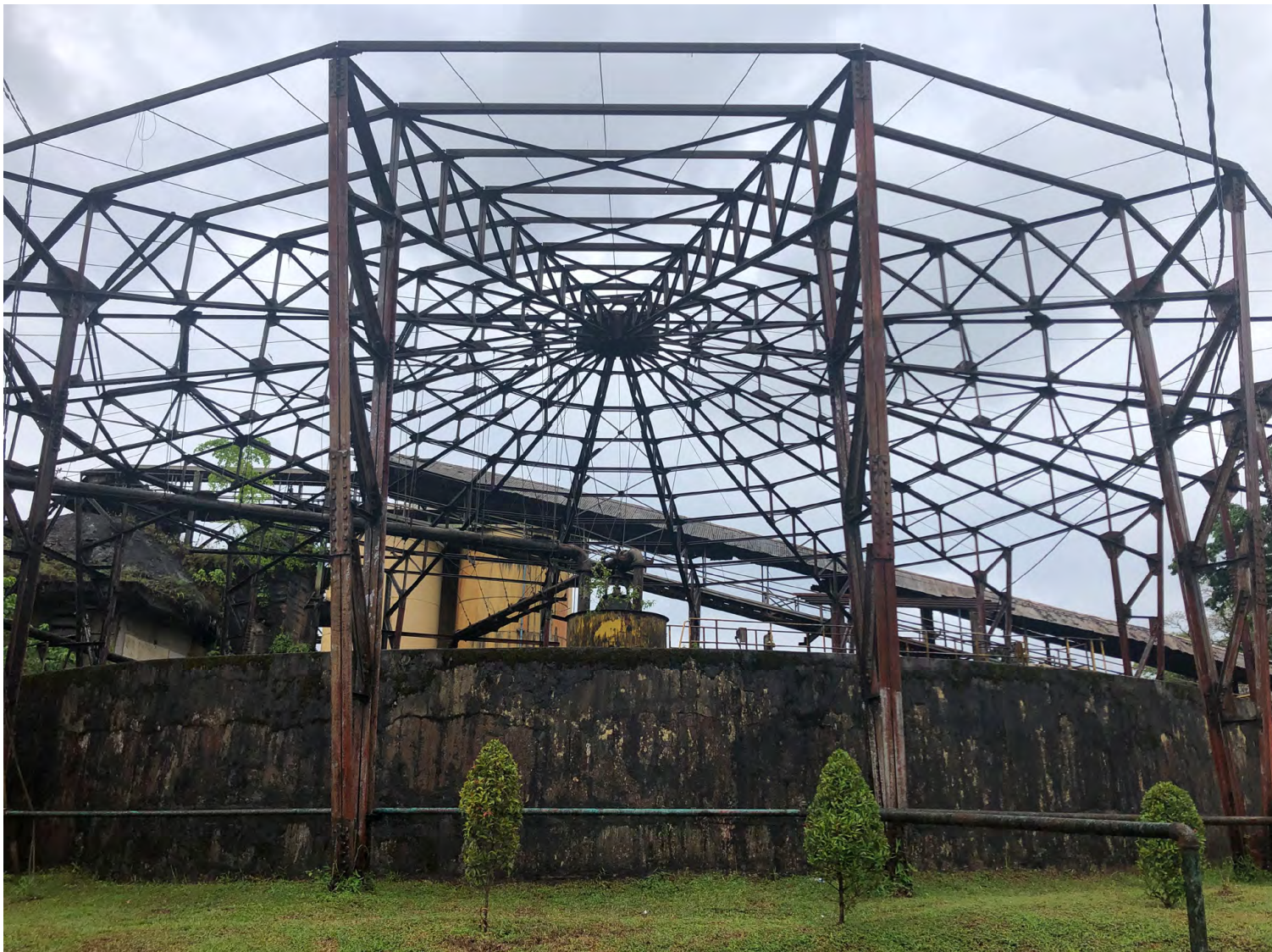
Cement plant of Indarung I in Indonesia (photo by author)
