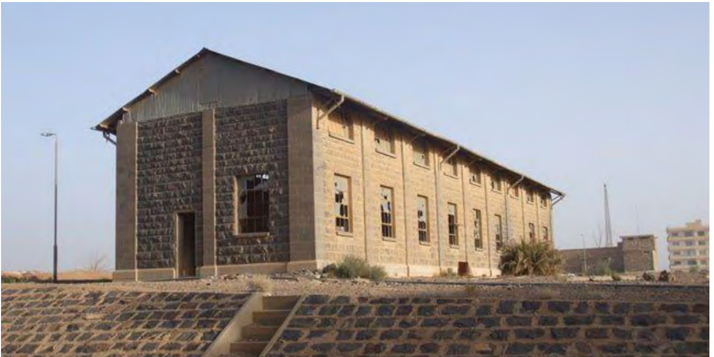
H5 Pump Station in Safawi, part of the IPC pipeline, was constructed in the 1930s using basalt stone (photo by Nader Atieh)
