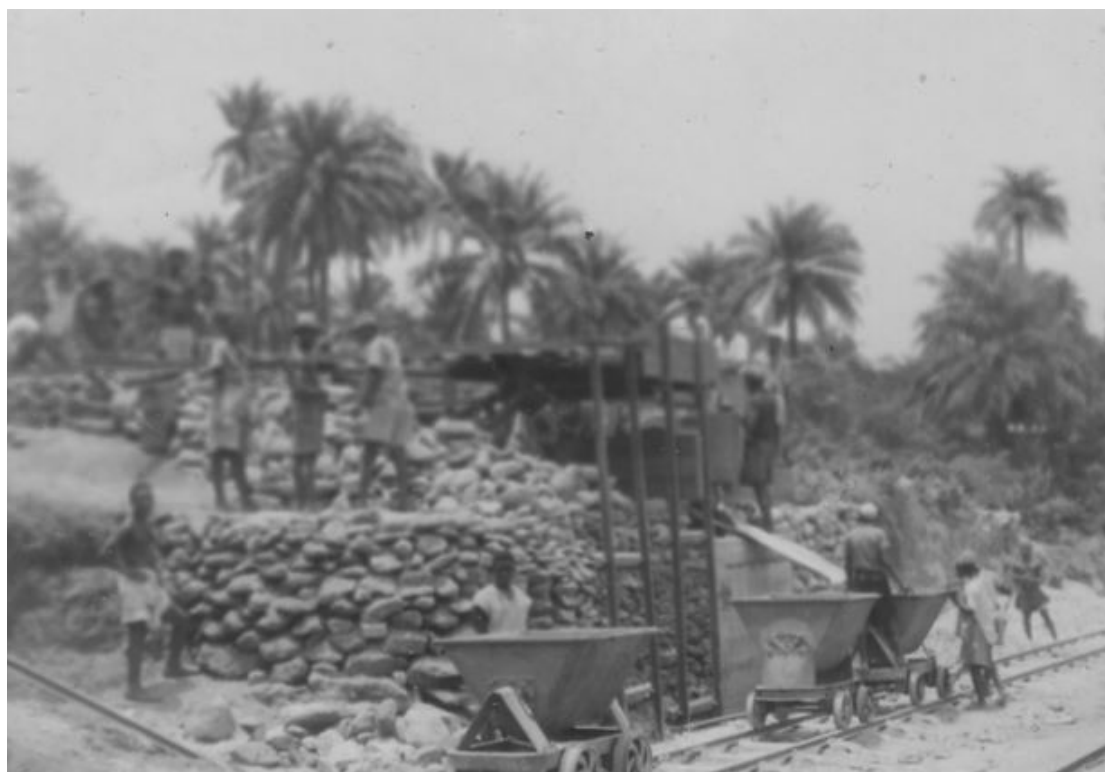
Hopper wagons being loaded with stone at Baoma Quarry, 1952 (photo provided by author)
