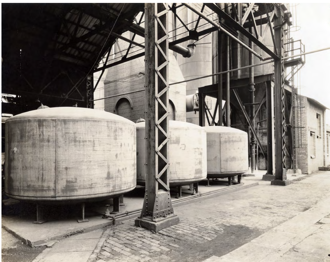
Scaife devices for water treatment for the boilers of the Power Plant, 1937. Monterrey, N.L., Mexico (DR. 46754 Nuevo León Photo Library – CONARTE, Fundidora Collection)
