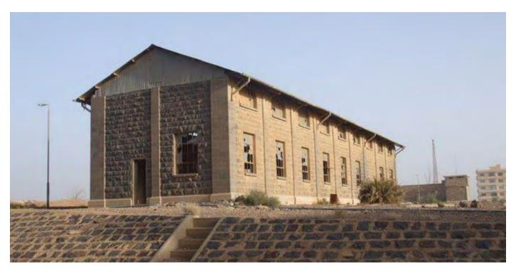
H5 Pump Station in Safawi, part of the IPC pipeline, was constructed in the 1930s using basalt stone (photo by Nader Atieh)
