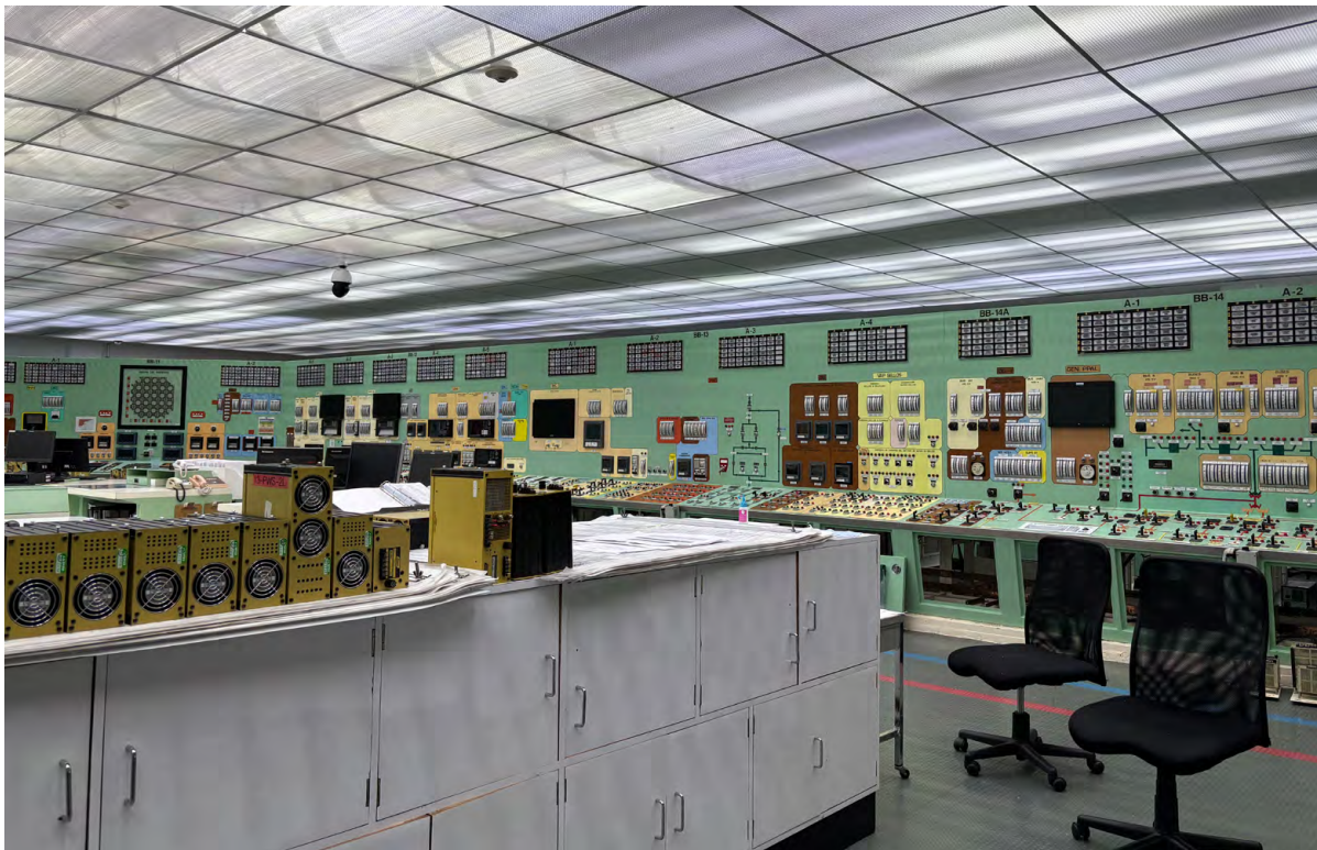
The reactor control centre simulator, a faithful copy of the control centre and where the new operators are trained (photo by author)
