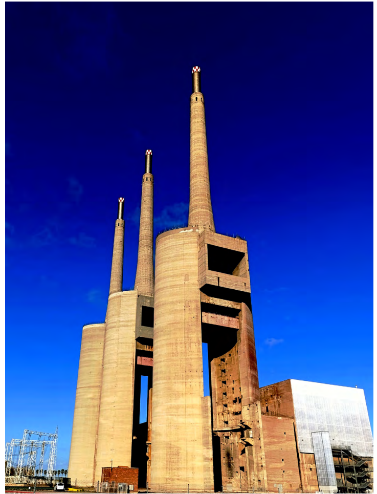
Concrete shells of the boilers and chimneys (photo by author)
