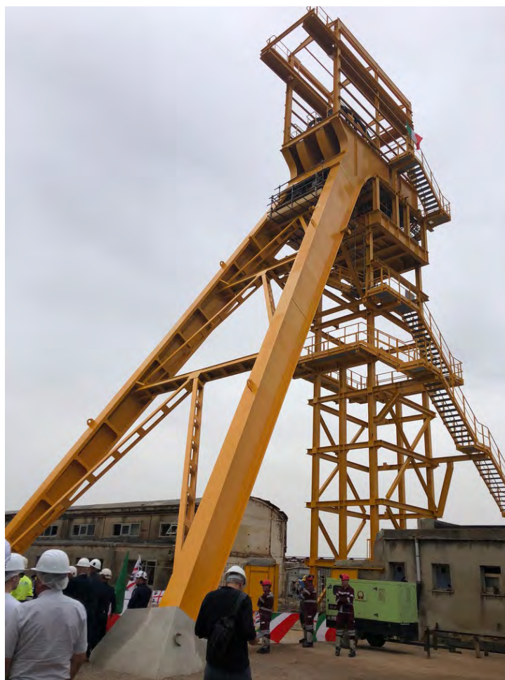
Shaft I extraction castle in Carbosulcis site, recently renovated (photo by AMA)
