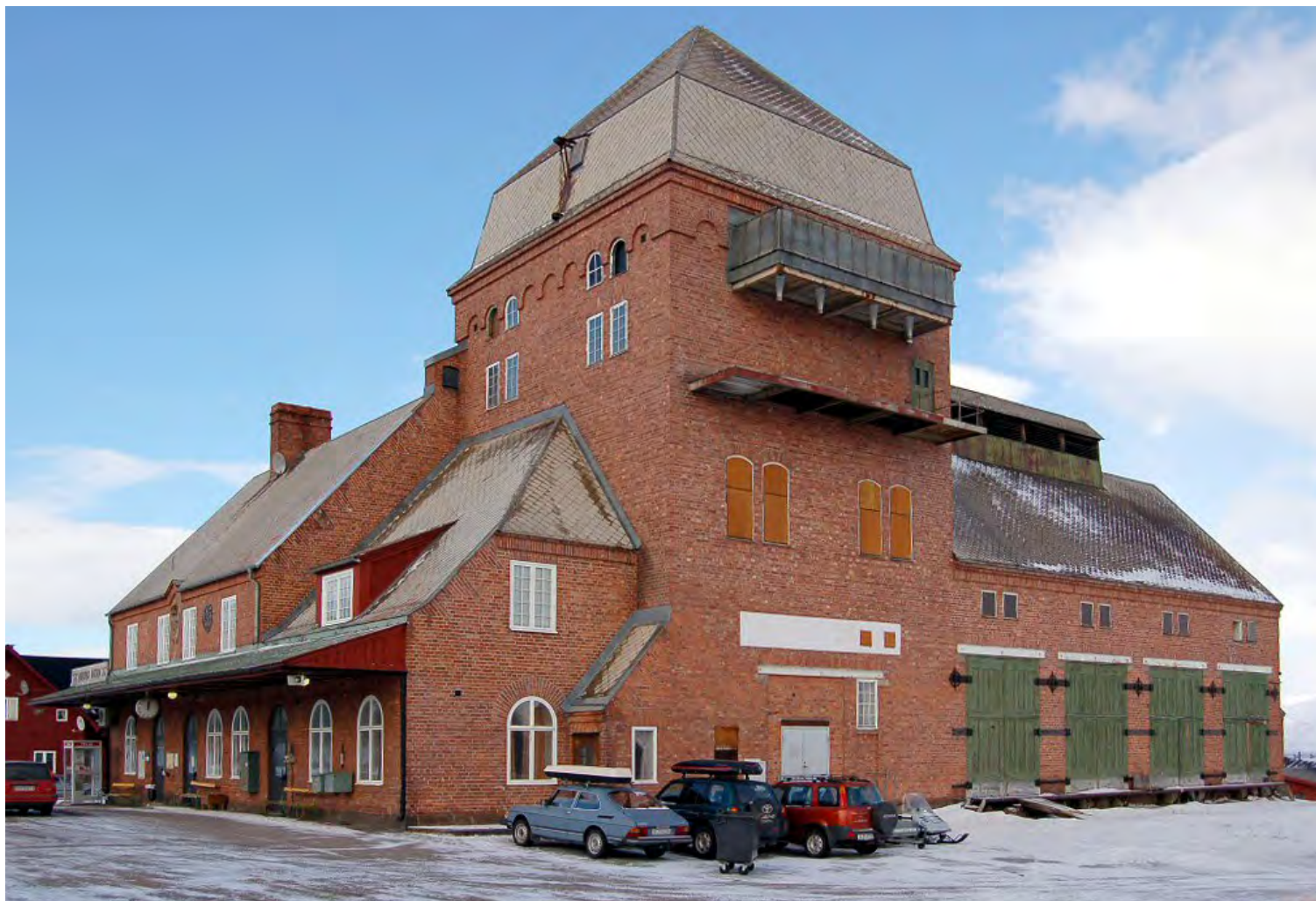
Torneträsk railway station. Built in 1915 as one out of four transformer buildings along the electrified Riksgränsbanan section (Kiruna to the Norwegian border) of Malmbanan (Iron Ore Railway) (photo by Curt Persson)
