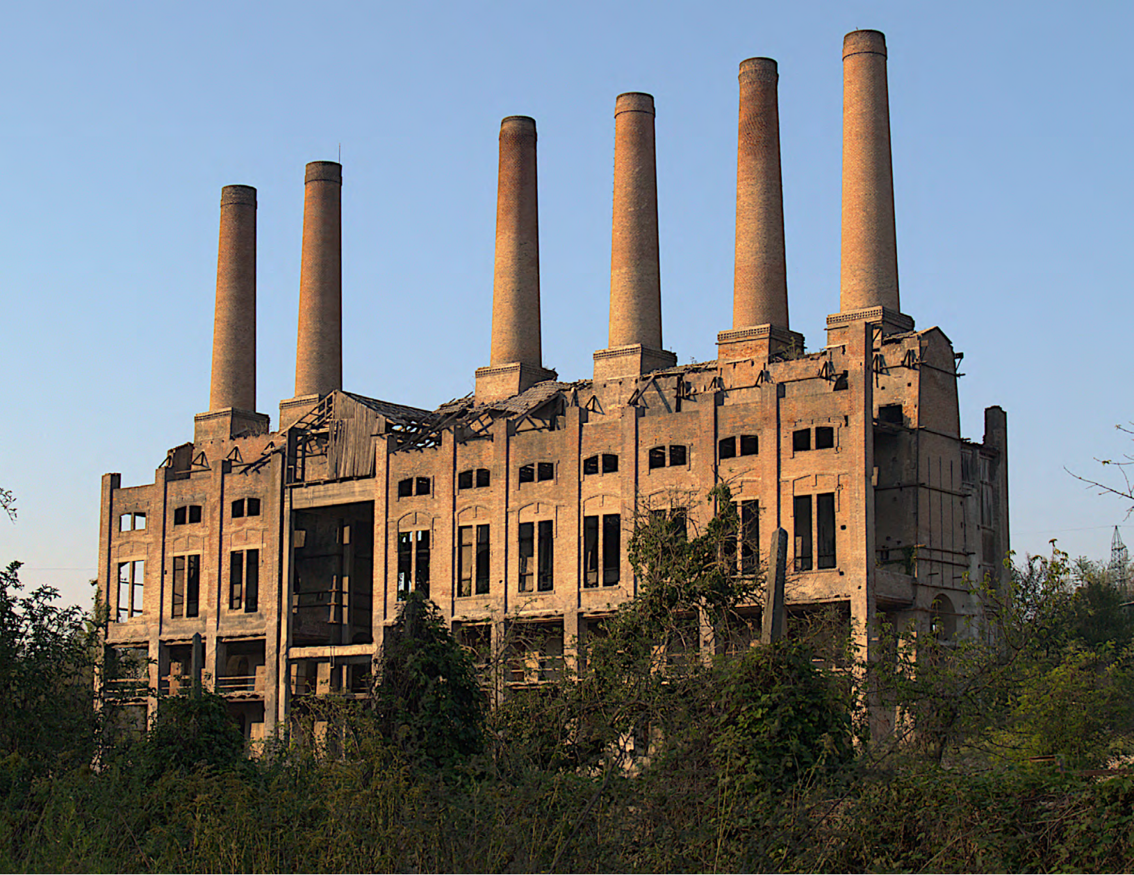
Cement Factory of the Società Anonima Milanese e Azzi, Ozzano Monferrato (Piedmont) A plant with six vertical kilns for the production of natural Portland cement, active between 1911 and 1924 September 2012
