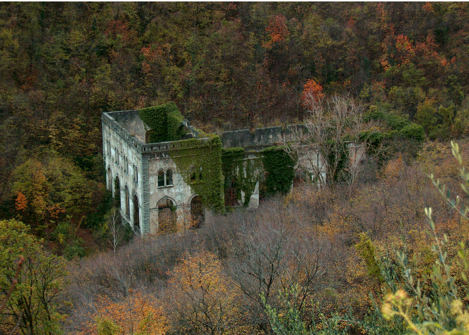
Biacesa Hydroelectric Power Plant on the Ponale Stream (Lake Garda, Trentino) A power plant supplying electricity to the city of Rovereto, operational from 1906 until the post-World War I period November 2007
