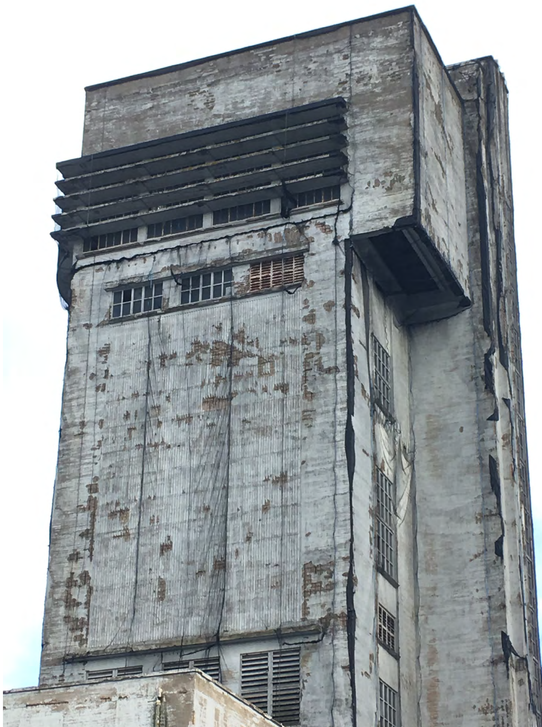
Shaft-tower of the colliery Saint-Albert in Péronnes-lez-Binche, a unique mine headgear in concrete, dating from the interwar period, threatened with demolition for many years (photo by Patrick Viaene, 2019)
