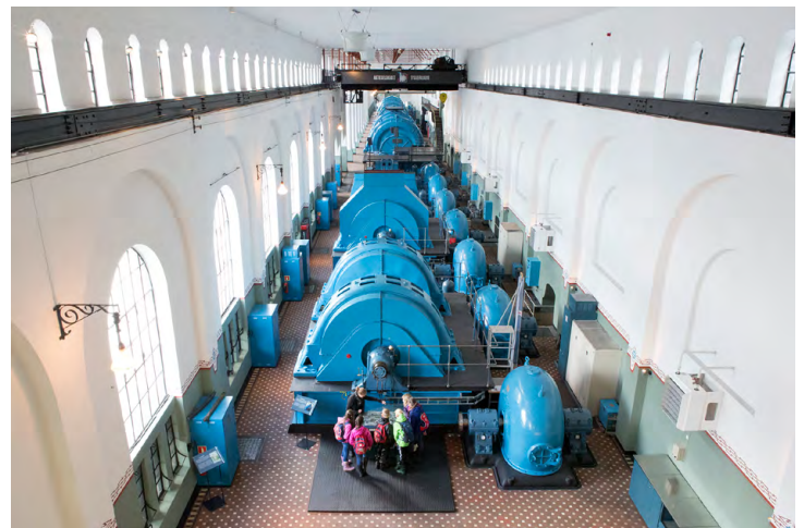
The Turbine Hall in the protected Tyssedal Hydropower Station, the main venue of Kraftmuseet (photo by Matt Coch)
