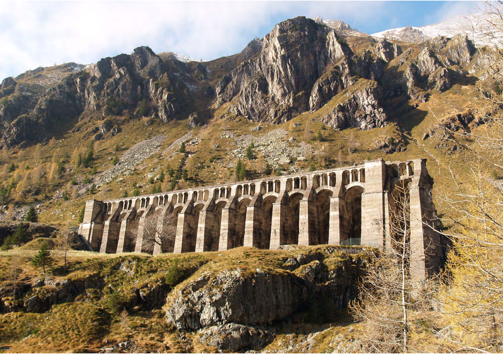
Gleno Dam, Vilminore di Scalve (Lombardy) A multiple-arch dam, initially planned as a gravity dam, built between 1919 and 1923. It collapsed on December 1, 1923, causing over 350 fatalities November 2013
