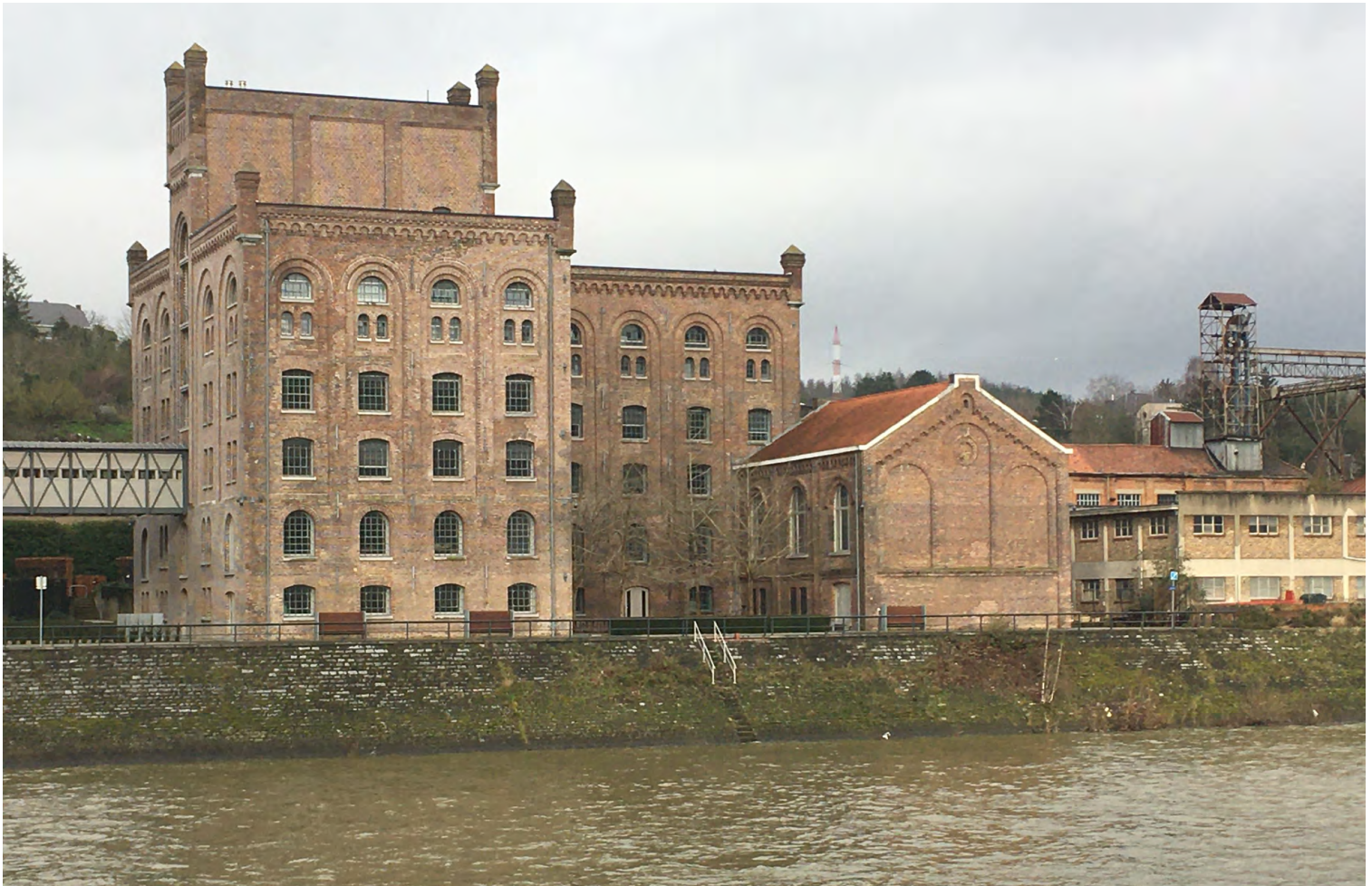
The 'Moulins de la Meuse', a former grain mill in Beez (Namur), reused as headquarters of the Walloon Heritage Conservation Administration, the location of the FABI-AWAP-PIWB symposium days (photo by Patrick Viaene, 2021)
