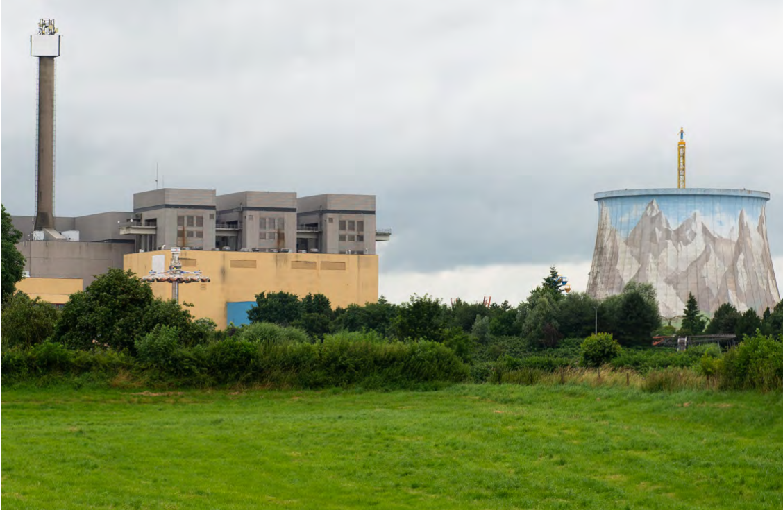
At Wunderland Kalkar in Germany, a disused cooling tower forms the centrepiece of a family theme park (photo by Bart Vanacker)
