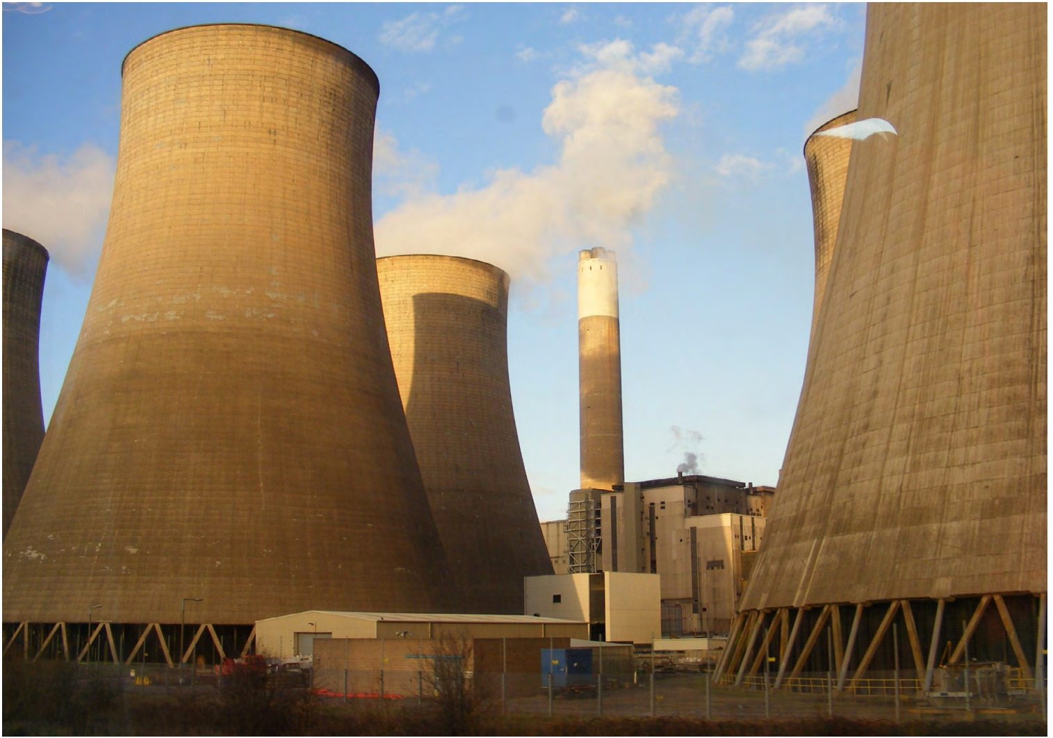
The last coal-fired power station, Ratcliffe-on-Soar, shut down on the 30th of September 2024 (photo by Mark Watson)
