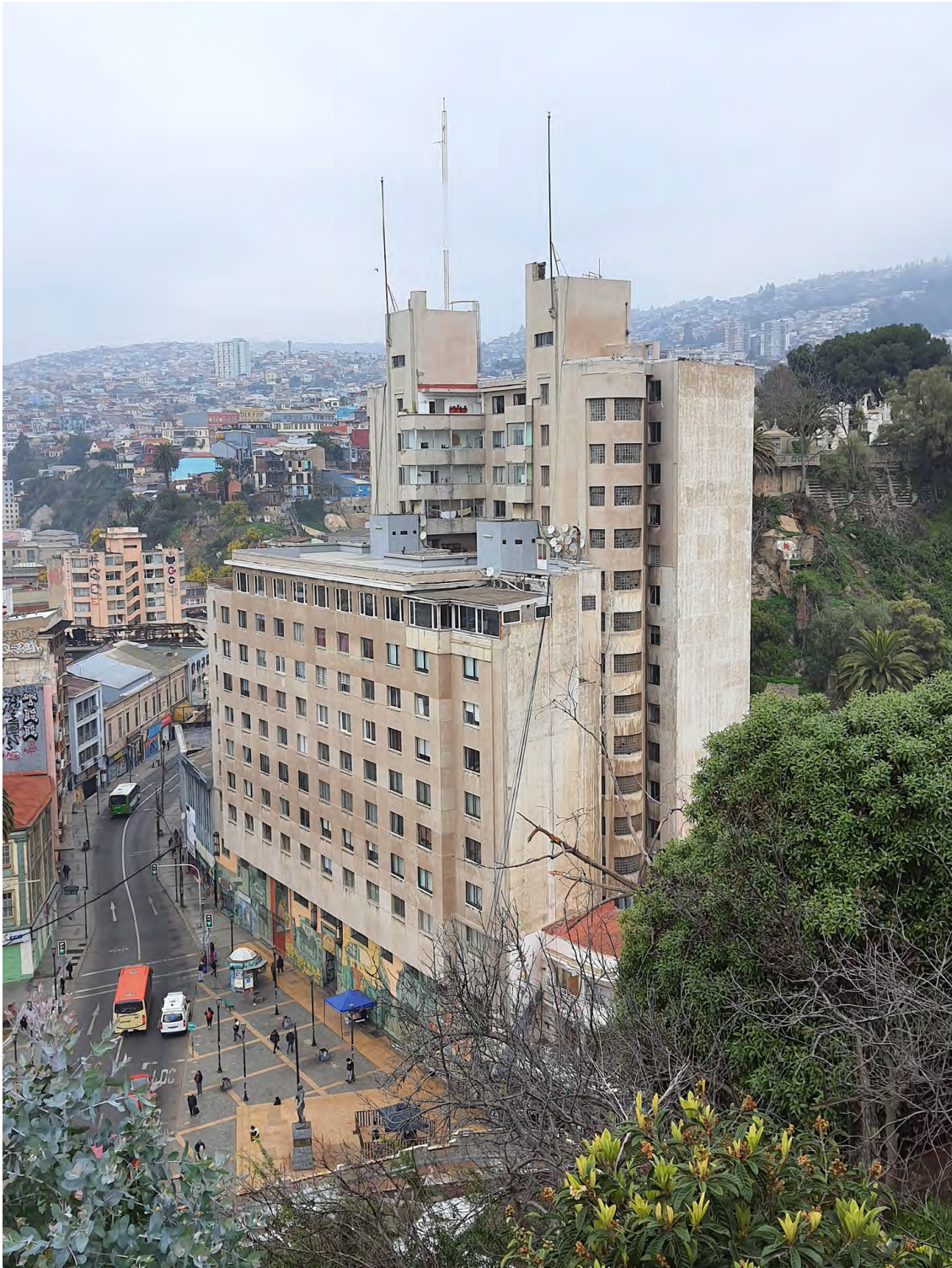
Valparaíso, Plazuela Anibal Pinto. The building is not only a beautiful example of “brutalist” architecture. It also is a counterweight to the cemetery behind it – a way to “repair” that seismically endangered hill (photo by author)
