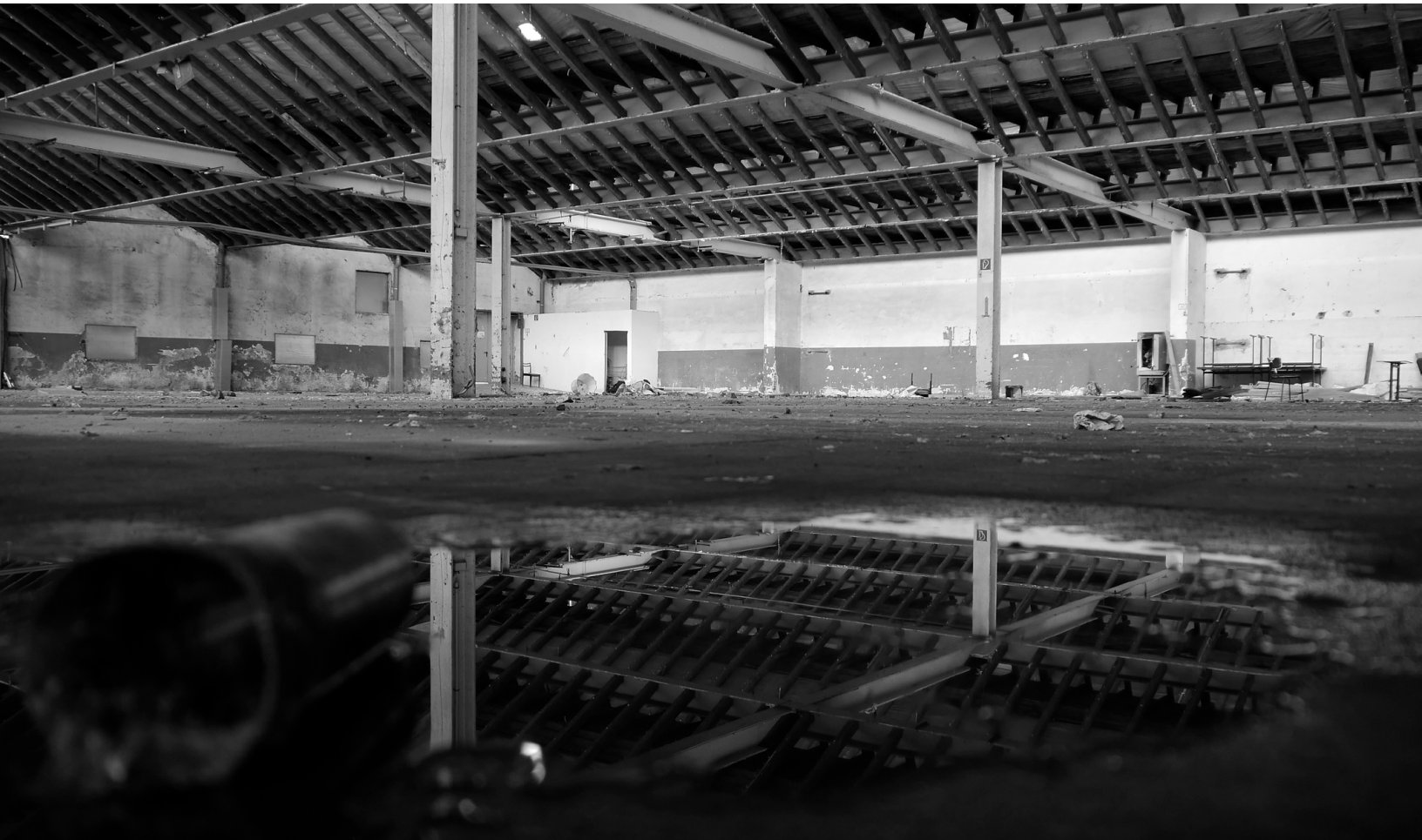
Roughing plant/Empty textile mill, Bocholt, Germany, 2020 (photo by author)
