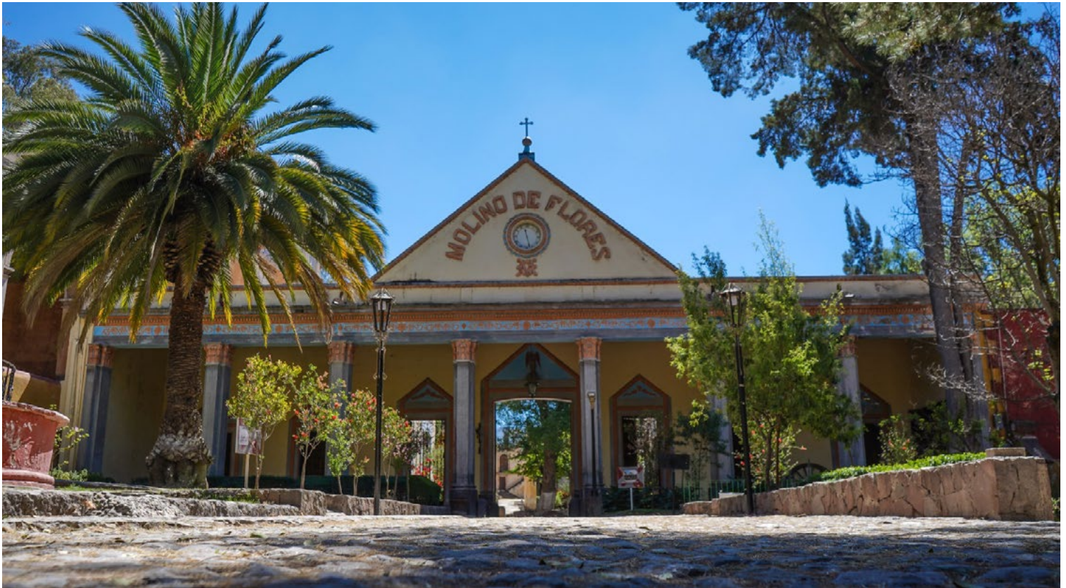
Main façade of the Molino de Flores (photo by José Luis Gonzalez Gonzalez)
