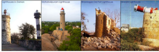
(L-R) The new Daman lighthouse is located near the historic lighthouse (1888) on the Mori Daman Portuguese fort the 26m high Mahabodipuram lighthouse constructed in 1902 using local granite is situated on a mound of stone close to the Chakrawarties temple Bhavnagar Old Fort Lighthouse severely damaged by earthquake in 2001, Mandi lighthouse was rendered unsafe due to an earthquake in 2001 and had to be pulled down. Courtesy: 'Indian Lighthouses', @gajwani (2000)
