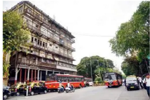
The Esplanade Mansion was constructed entirely from pre-fabricated cast-iron in 1865
