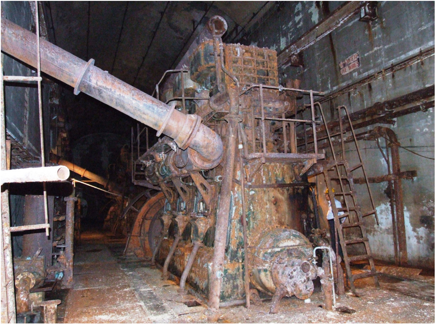
One of only 115 General Electric Fullagar generating diesel engines, in the Kordin power station.
