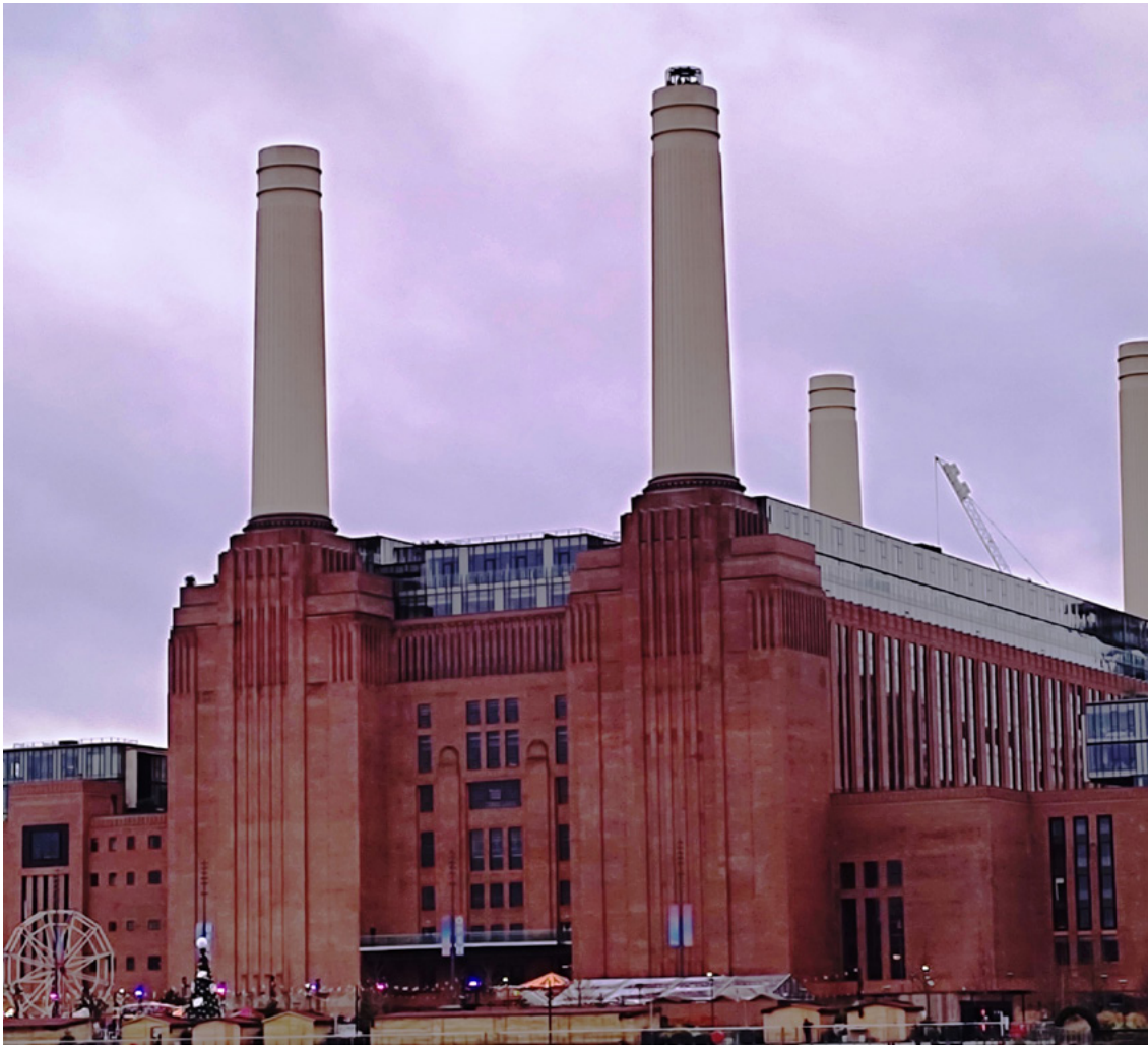
The power station as completed, new windows cut through the brickwork and the glass-walled apartments in the space between the chimneys.
