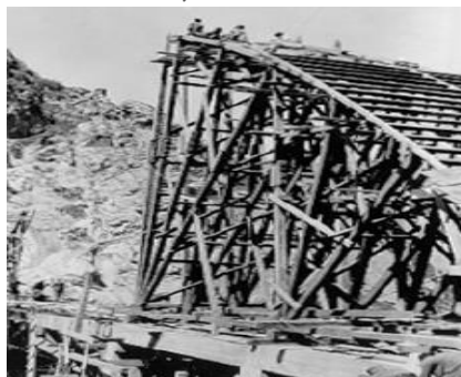
Completing the arc slab molds
