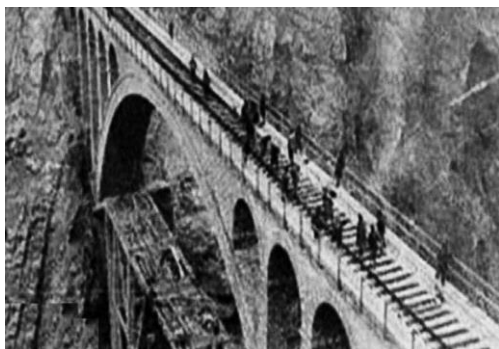
Traversing and railing operations
