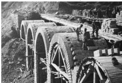
Installing arc slab molds
