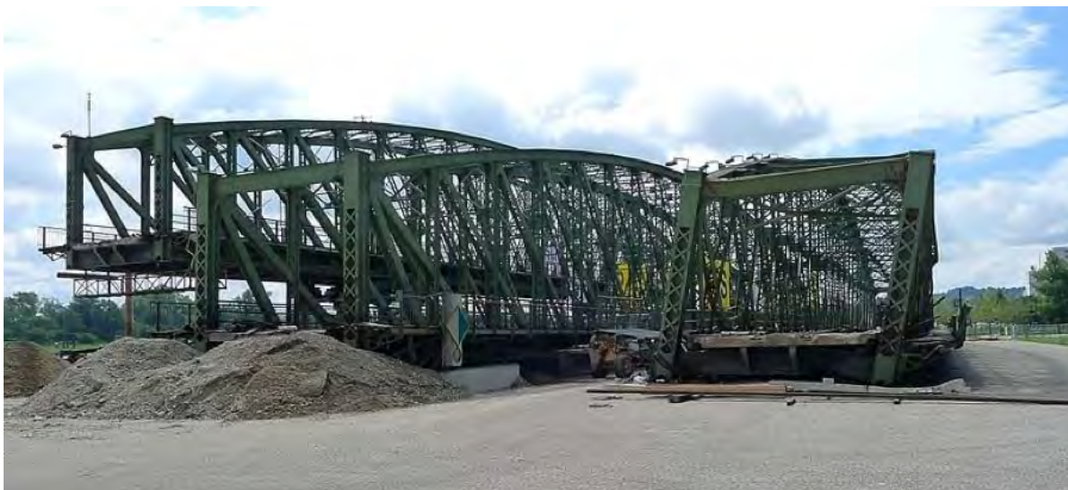
Scrapping of the rail/road-bridge across the Danube in the city of Linz. Photo: Bernhard Holub (CC BY-SA 3.0, from Wikimedia Commons)
