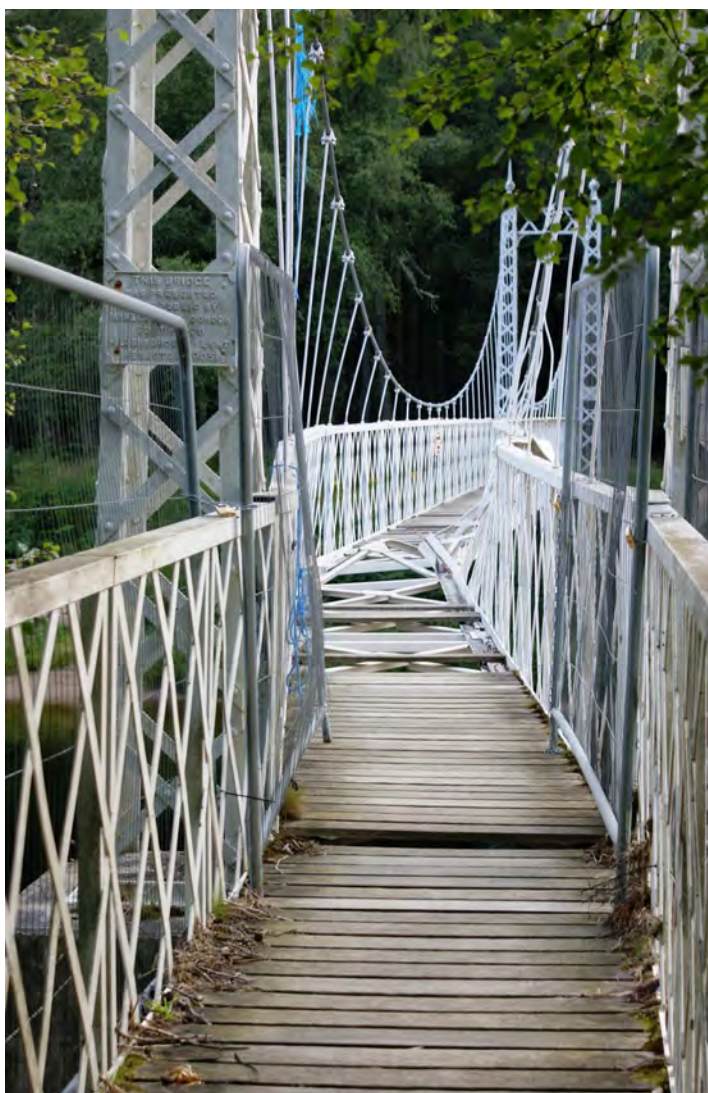
Cambus o'May Suspension Bridge, Aberdeenshire, damaged by floods in 2016 © Mrak Watson
