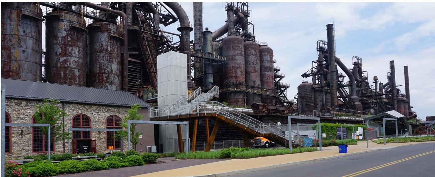
The former Bethlehem Steel blast furnaces.
