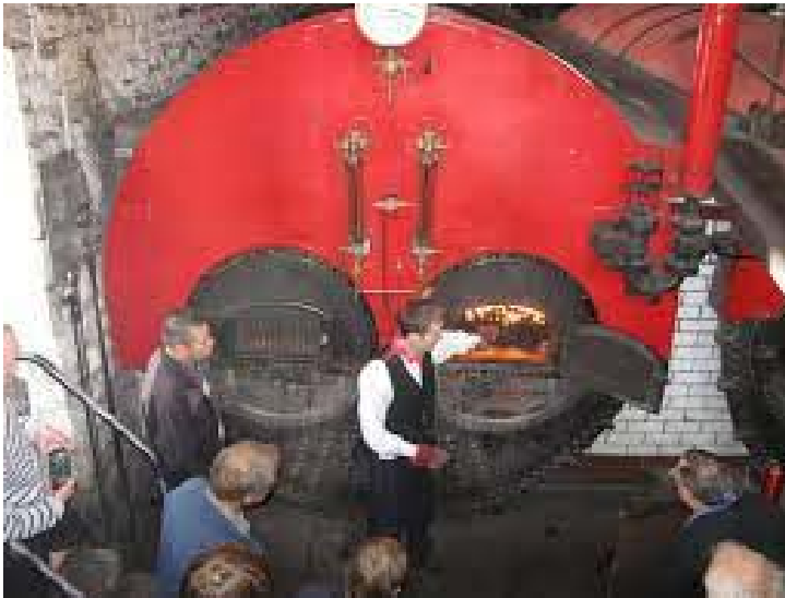
Visitors feel the heat of a stoker firing one of the Lancashire boilers in the Queen Street textile mill near Burnley, Lancashire. Creative Commons
