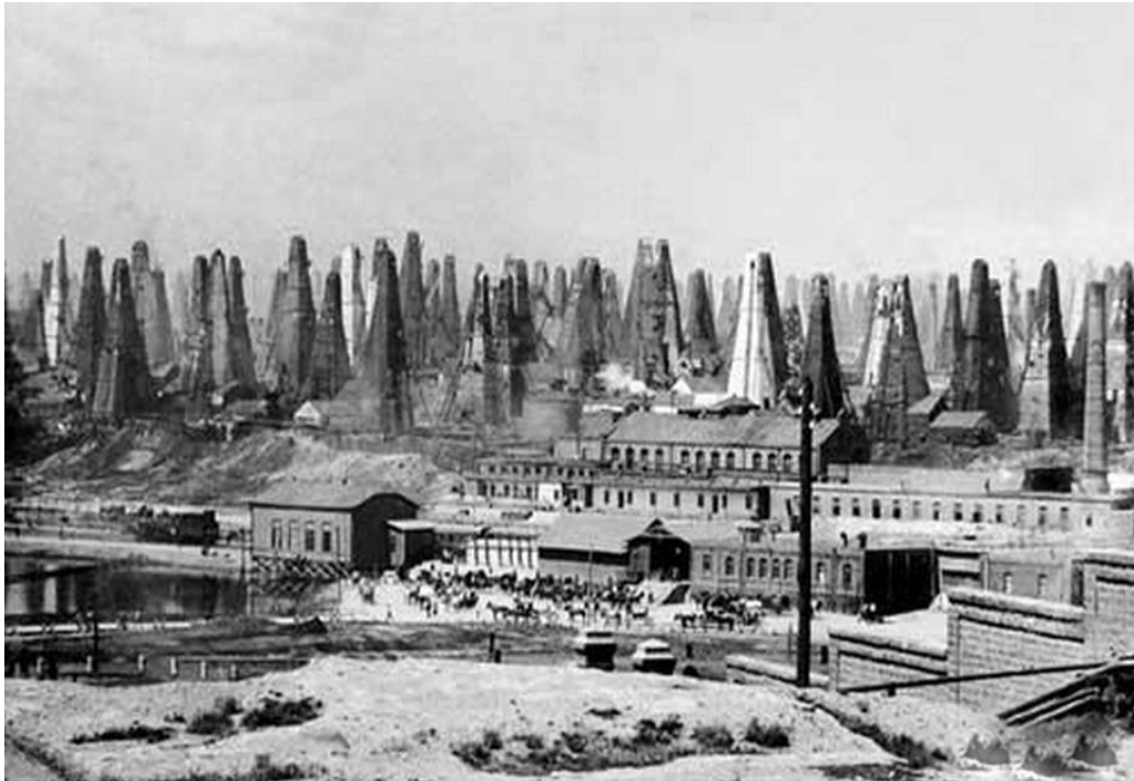
Derricks encased in wooden shuttering of the Nobel Brothers Petroleum Company, Branobel, in Balakhani, Baku c. 1890 (© Wikipedia Commons).
