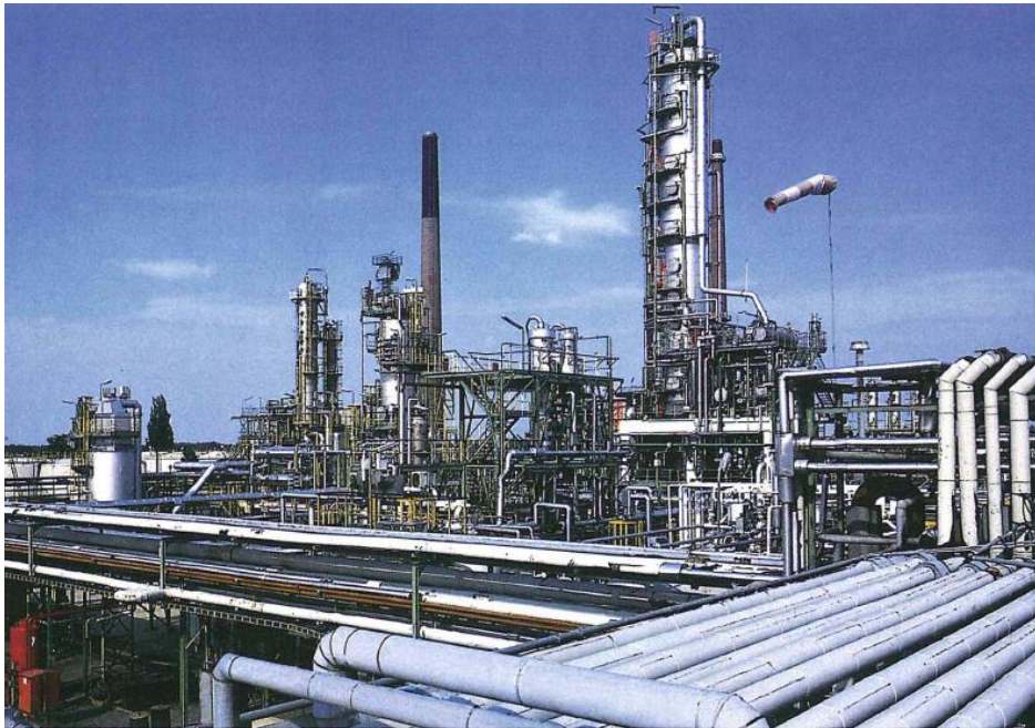
Two images of the Salzbergen refinery from 1903 and 2010 illustrate how radically these plants have changed (© Oehlke 2010).
