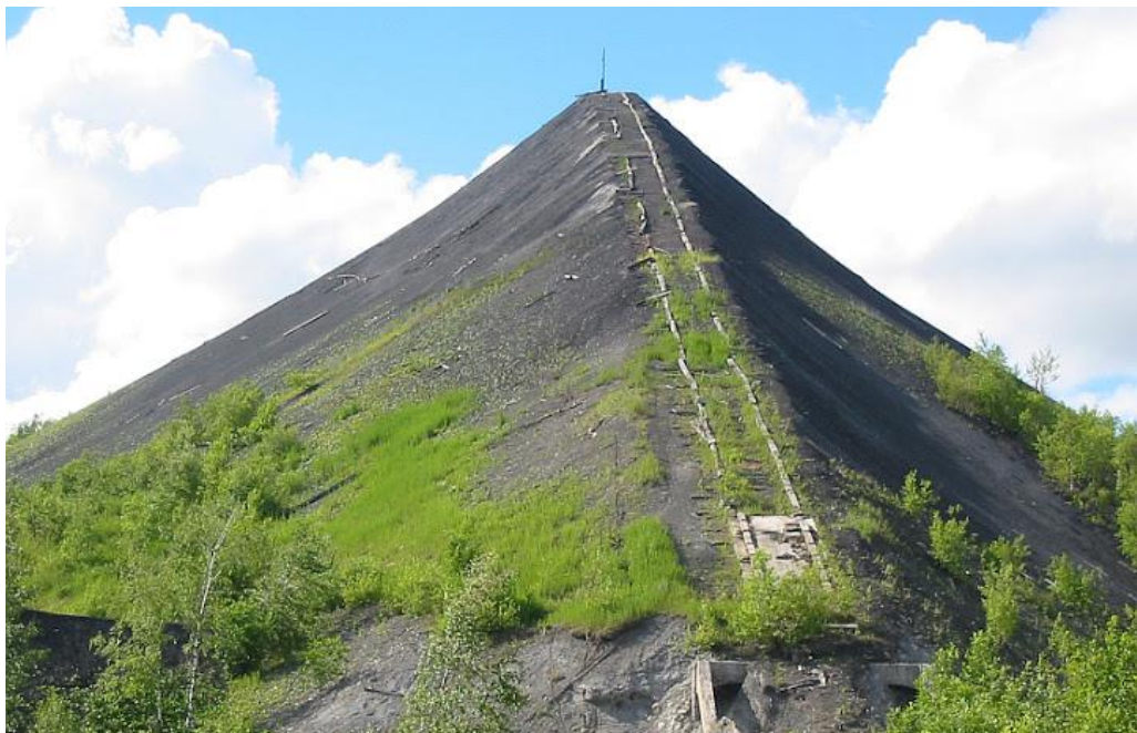
A waste heap in Estonia with remains of an inclined plain, formed from extracting shale oil from oil shale. (© Siim Sepp)
