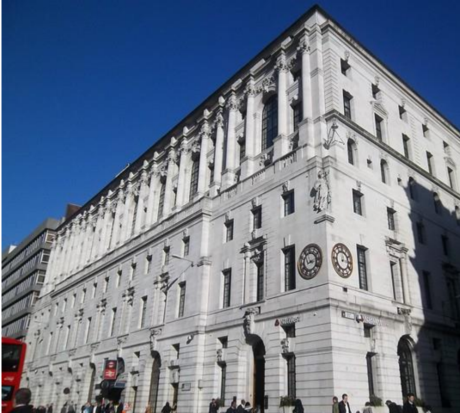
The Anglo-Persian Oil Company commissioned the favourite architect of the British Empire, Edwin Lutyens, to build its London office. (© Jamie Barras)
