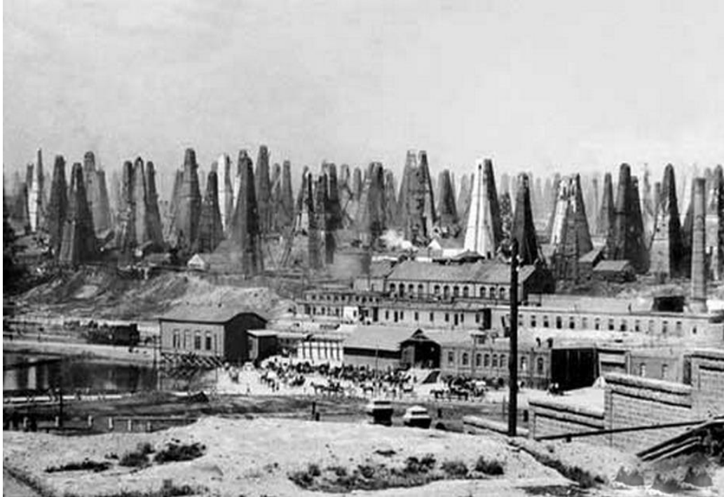
Derricks encased in wooden shuttering of the Nobel Brothers Petroleum Company, Branobel, in Balakhani, Baku c. 1890 (© Wikipedia Commons).
