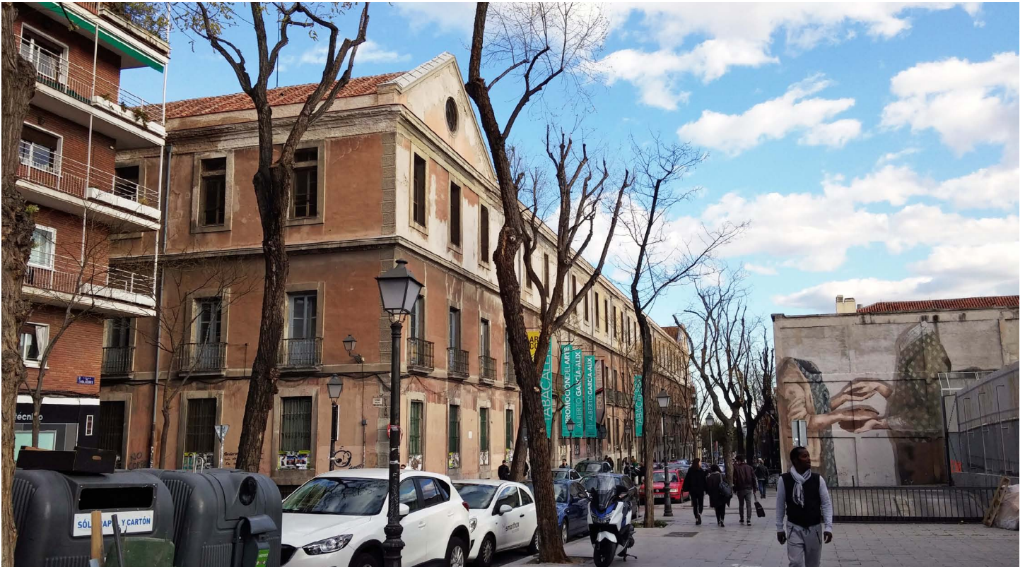
The Madrid tobacco factory has been partially reconverted into an exhibition space and social centre. (Carolina Castañeda, 2016)
