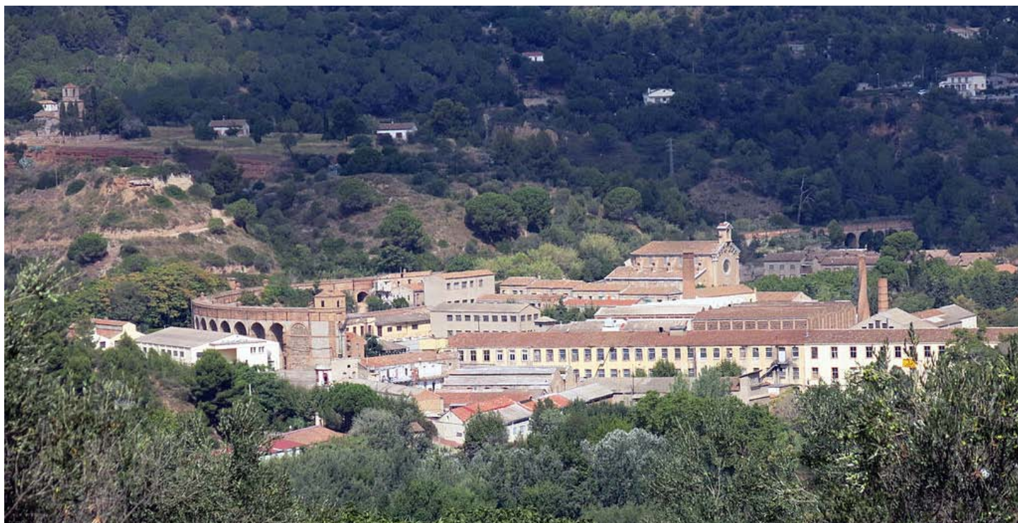
Participants visited the archetypal Catalan textile village, the Colònia Sedó. This view shows the aqueduct which brought water for the turbines on the left, the factory in the foreground with the church behind. The unique spiral chimney can also be glimpsed. Photo: Creative Commons.
