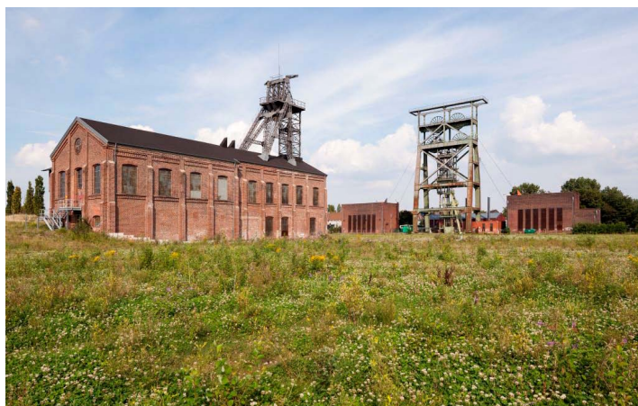
Gneisenau colliery shaft 2 and shaft 4 in Dortmund with the Tomson Bock built in 1886 (left) and the Doppelbock frame built in 1933/34 (right). Photo: Werner Hannappel, 2015.
