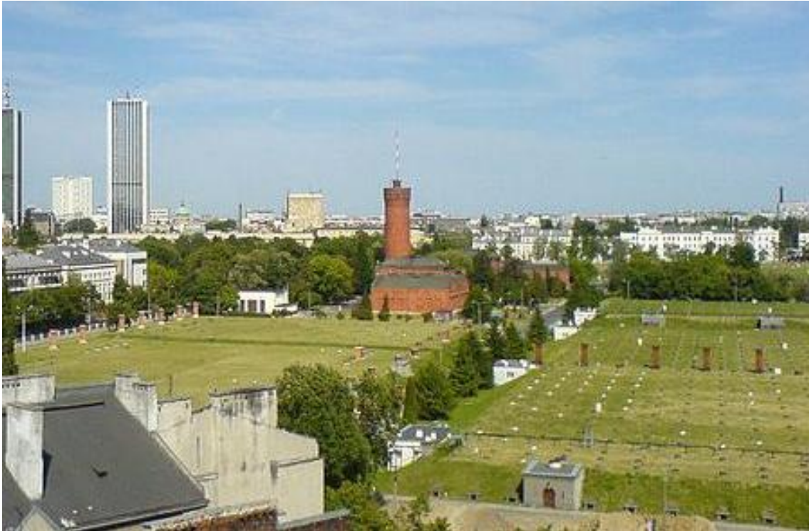
Filtry Lindleya (Lindley's Filters) opened in 1886 to distribute filtered river water in Warsaw. Named after the prolific water engineer William Lindley, it includes a group of slow sand filters, covered reservoir, pumping station and water tower. (Creative Commons)
