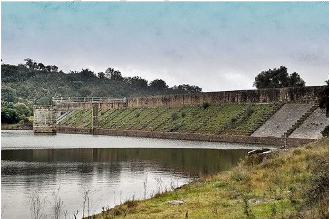
The Cornalvo gravity dam supplied water to the Roman city of Mérida in Spain from the second century CE. Charly Morlock via Wikipedia Commons
