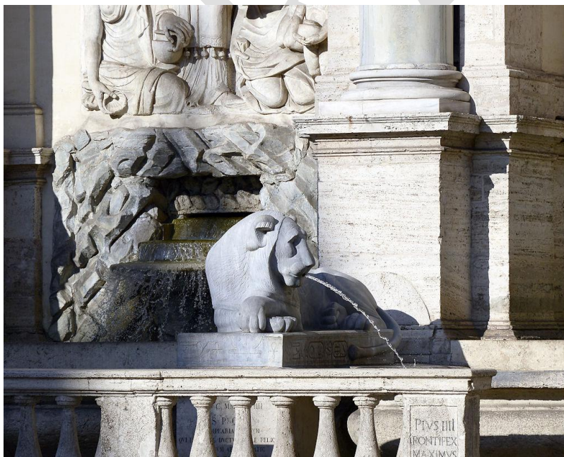
Public fountainheads like the Fontana dell'acqua Felice were part of the Counter Reformation renewal of the water supply system in Rome. Wikipedia Commons
