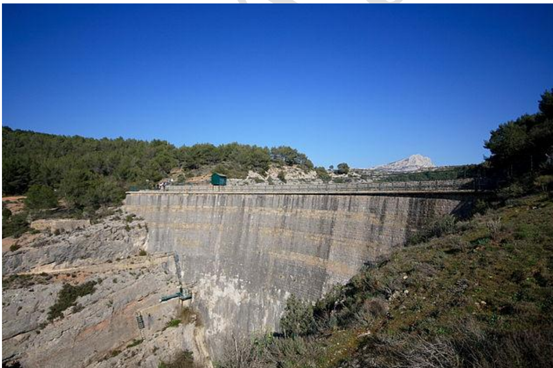
The Barrage Zola is an early masonry arch dam built to provide Aix-en-Provence with safe water following a cholera epidemic in the city. (Creative Commons)
