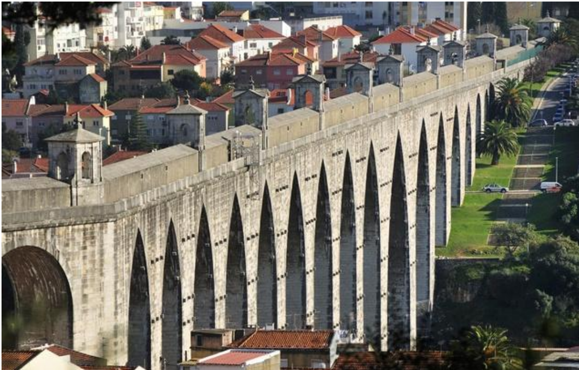
Alcântara aqueduct bridge. (Wikipedia Commons)
