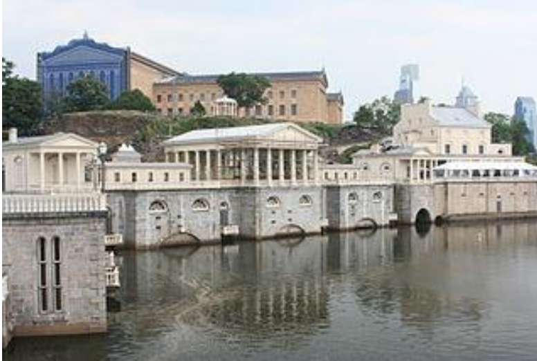
At the Fairmount Water Works on the Schuylkill river in Philadelphia, water wheels replaced beam engines to work the lift pumps. Ben Franske, Creative Commons
