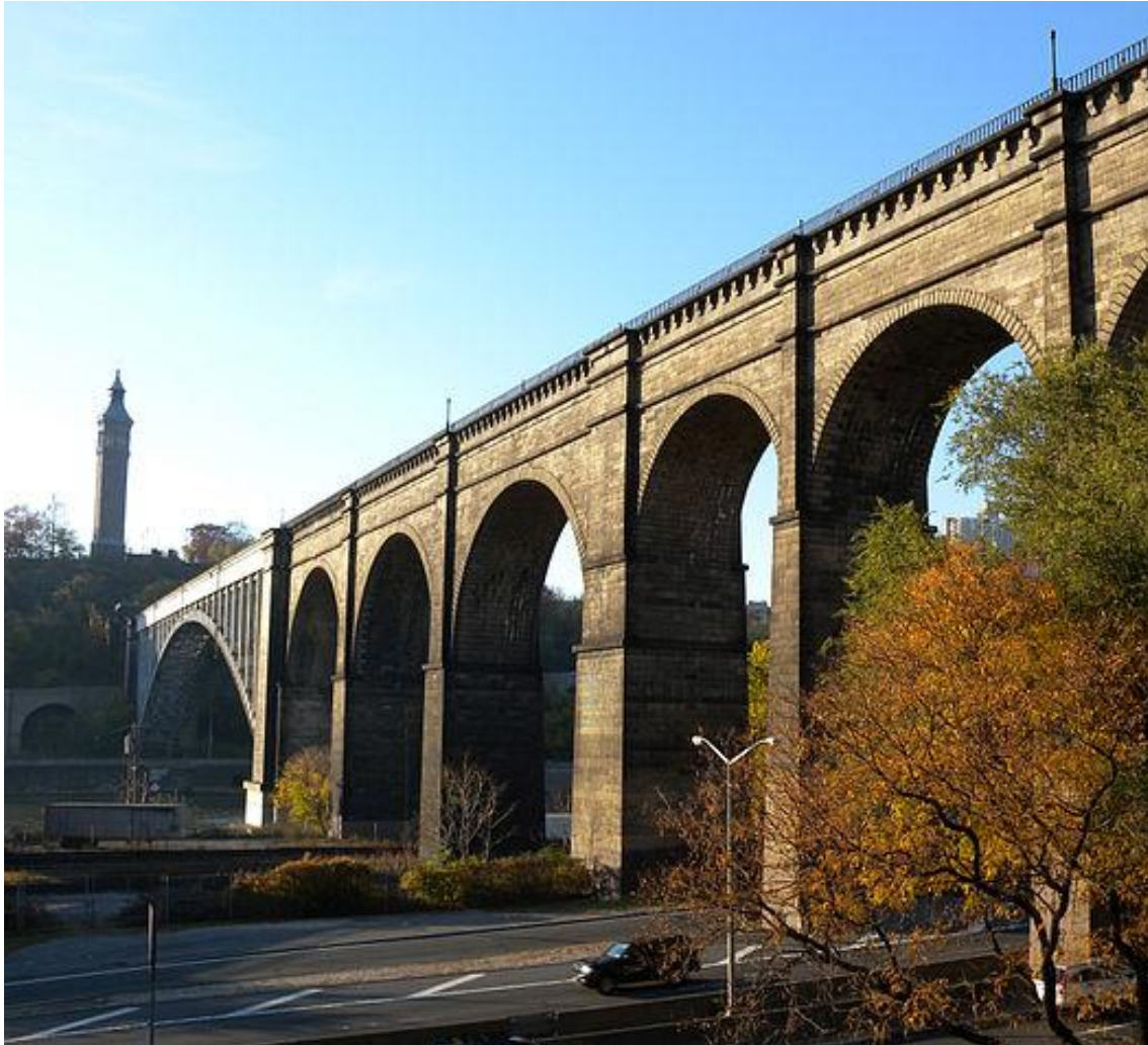
The 1837-48 High Bridge entering Manhattan. Most of the masonry arches were replaced by the 1927 steel arch. Jim Henderson, via Wikimedia Commons
