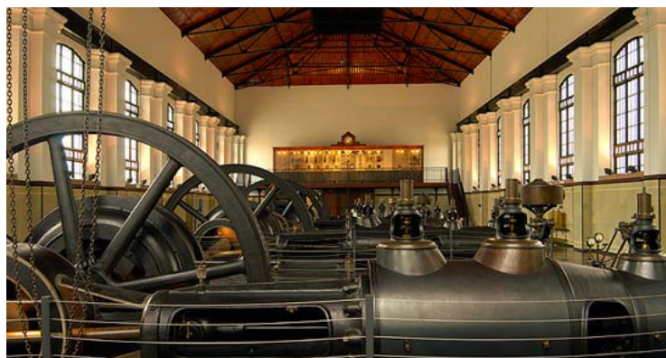
Fives-Lille steam pumps in the 1905 pumping station which is now the Museu Agbar de les Aigües. © MAA
