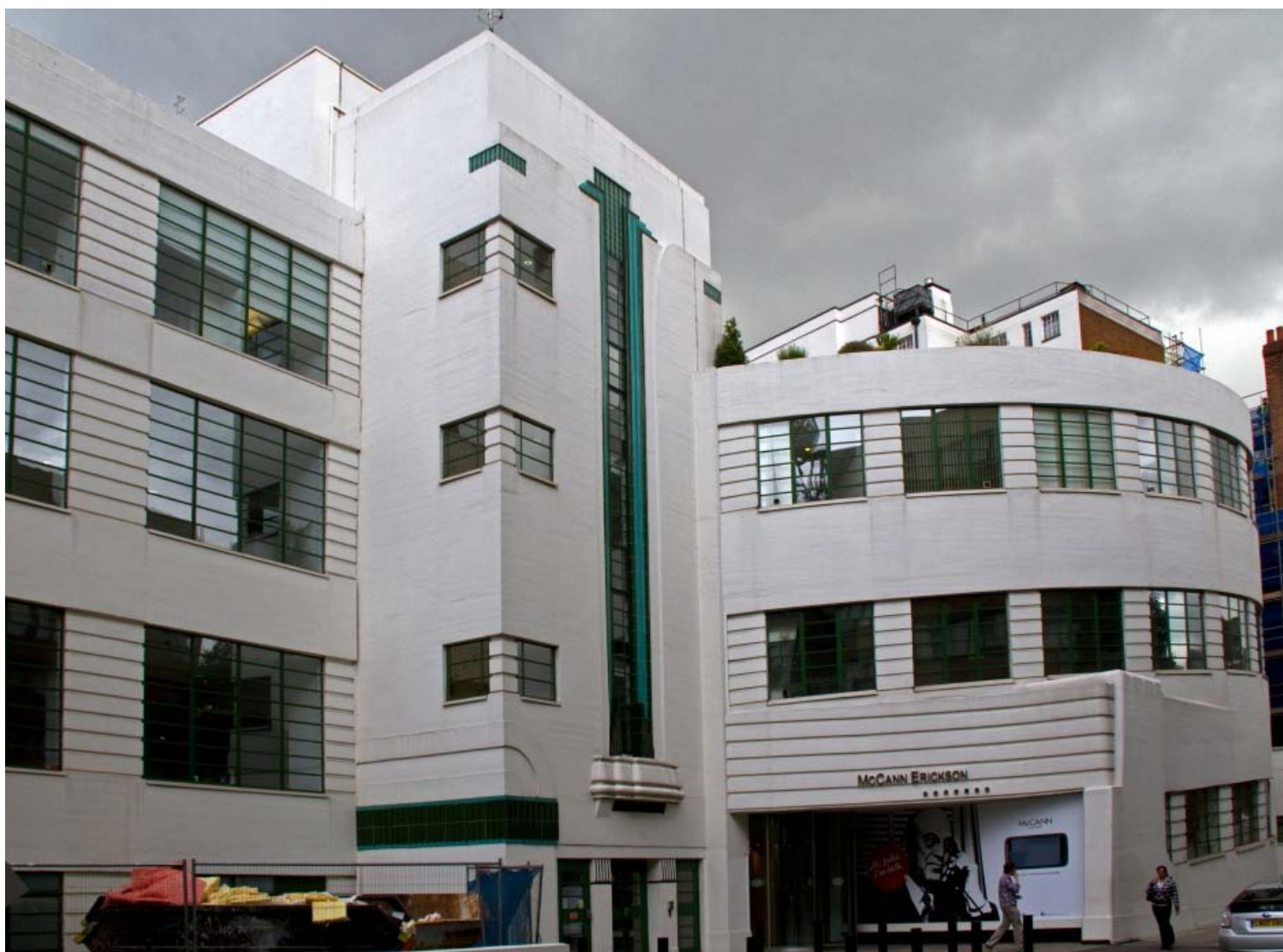
The Daimler Hire Garage, London, (1931; Grade II) by Wallis, Gilbert and Partners. Upper storeys provided parking reached by a spiral ramp which gave the building its unique appearance. © Tony Hisgett, via Wikimedia Commons
