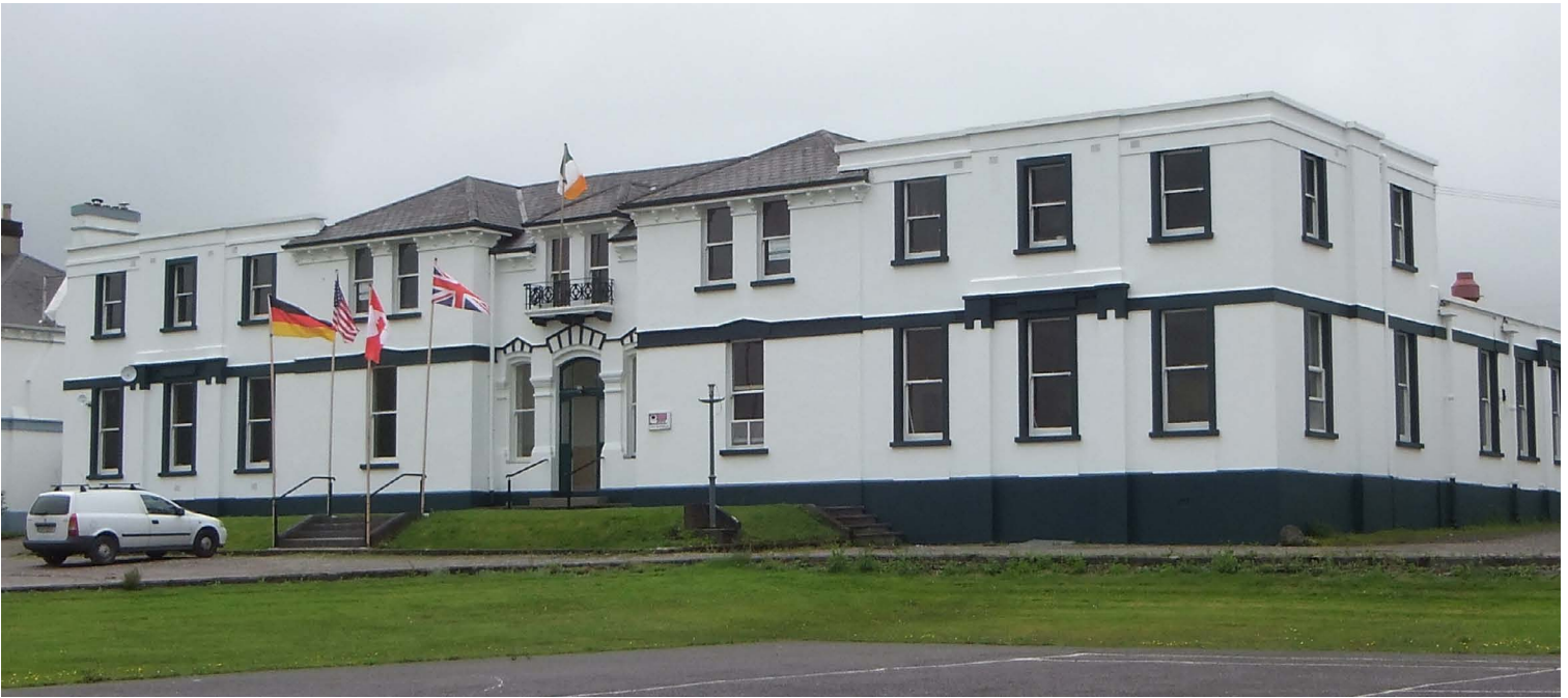
The 1868 cable station building at Valentia, Ireland
