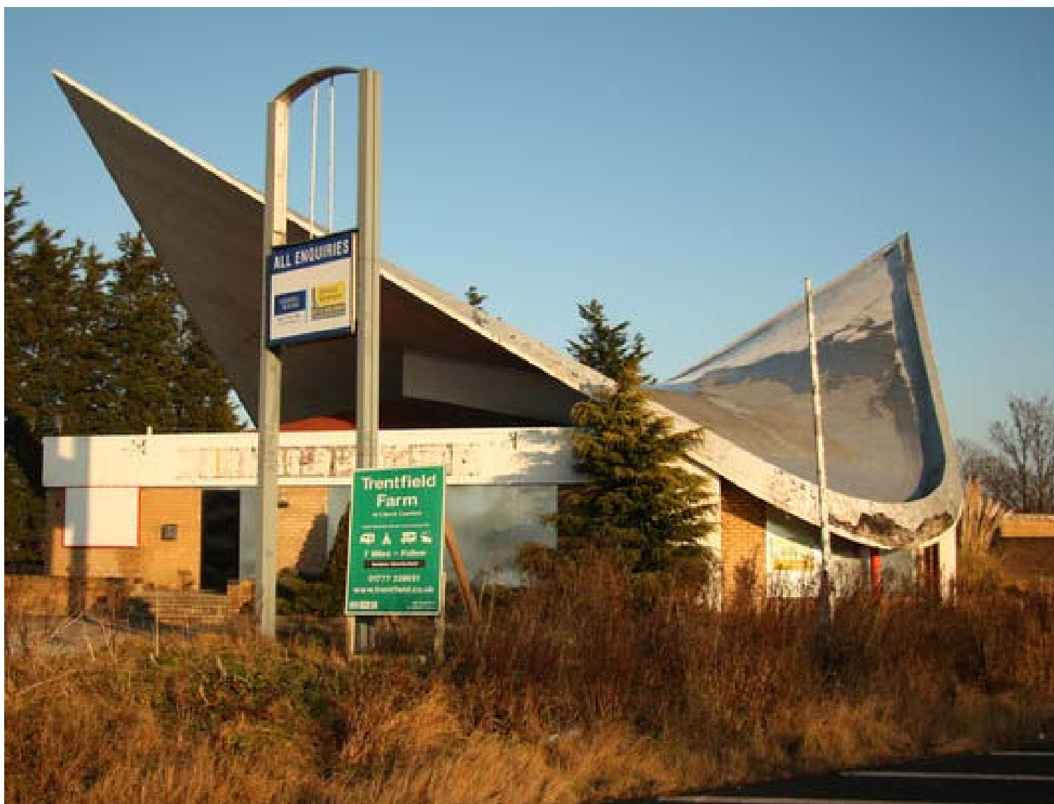
Markham Moor petrol station with its innovative hyperboloid concrete shell canopy (c.1960-61) was converted to a roadside restaurant in the 1980s. © Richard Croft, via Wikimedia Commons
