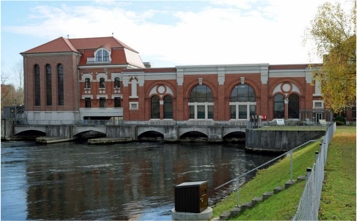
Hydraulic electric power station on the Lech canal from 1906.
