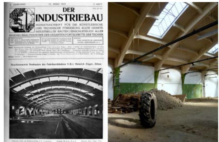
Industrial hall of the former Matador factory designed by the German architect Heinrich Ziegler, built in 1912, on the front page of the Der Industriebau from March 15, 1919 (Source: Research Centre for Industrial Heritage FA CTU Prague). On the right, the interior of the building today (Photo: Silvia Slaničková).
