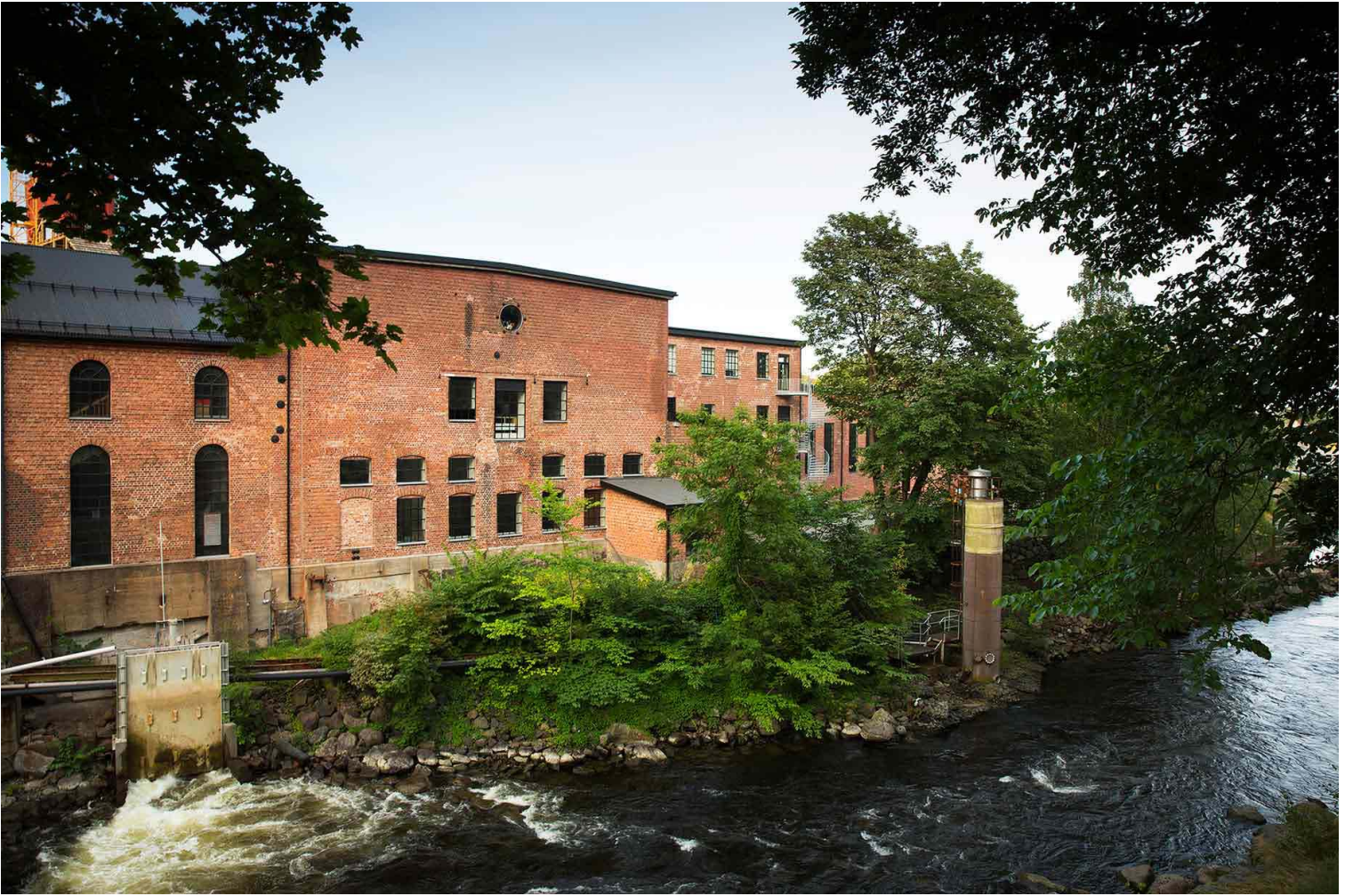
The Hammerdalen mill was used for processing raw wood into wood pulp, cellulose, cardboard or fibreboard. It was constructed in 1875 and extended in 1905 and 1975, and finally closed down in 2000. It was totally renovated and adapted for the Larvik Cultural School and the dance studio Nille in 2007/2008. Photo: Fritzøe Eiendom AS
