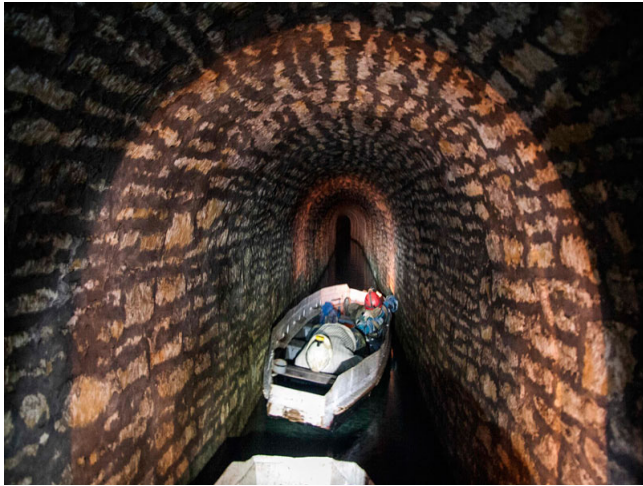
Friedrich Deep Adit, close masonry arched tunnel lining, typical of a great many kilometres that still function in the purpose for which they were constructed almost two centuries ago.
