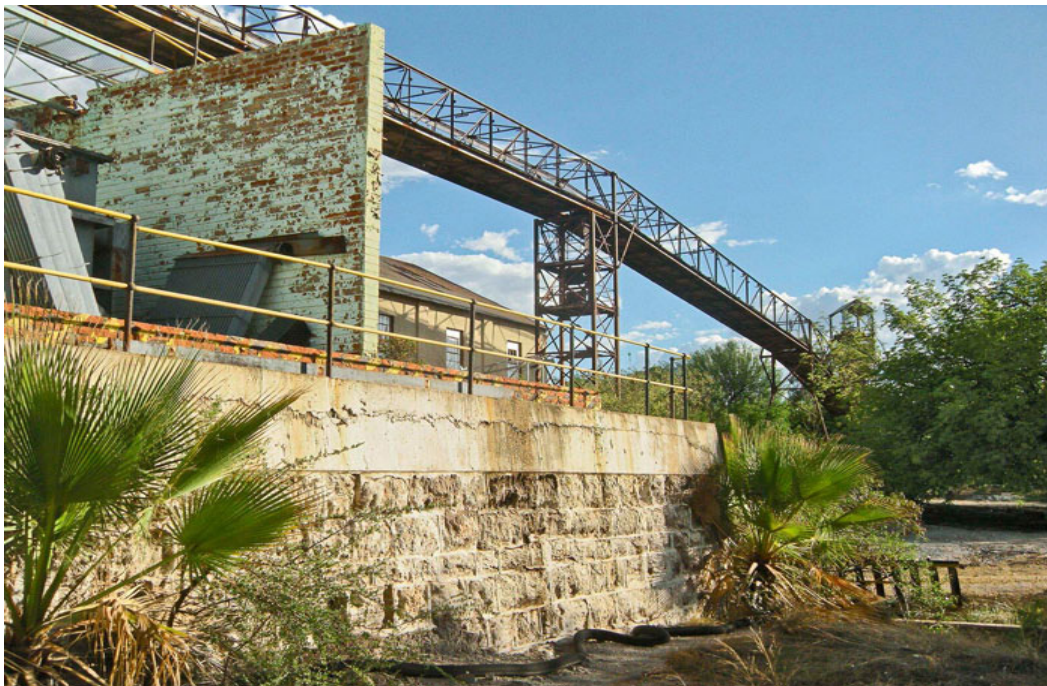
The horizontal conveyor from the Friedrich-Wilhelm-shaft was about 200 meters long, about 100 meters are in good condition.
