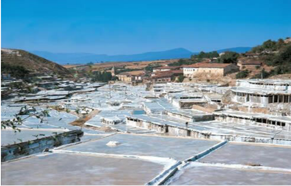
Valle Salado: Salt has been produced here continuously for over 6,500 years. Wooden channels transport the salt water on to evaporation terraces built of dry stone, wood and clay.
