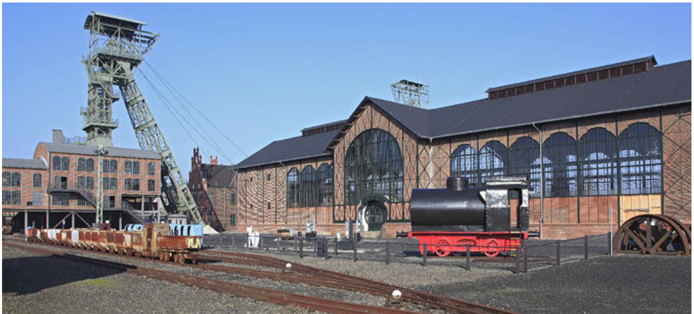
Erected in Dusseldorf for the 1902 Industrial Exhibition, the hall was dismantled and moved 100 km to Dortmund where it was re-erected with the famous Jugendstil entrance.
