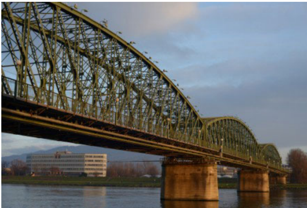
The bridge combined three lattice-girder bridge segments with curved top boom and 83 m span each for crossing the river; accompanied by four lattice-girder bridge segments with parallel top boom and 26,6 / 36,3 m span each.
