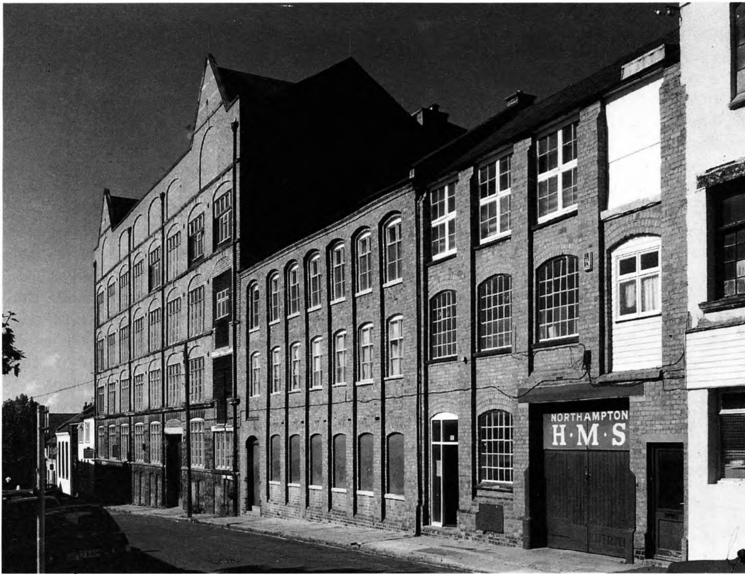
Figure 4. Church & Co.'s extensive former factory in Duke Street, Northampton. The original seven-bay factory of 1874 is in the centre; to the right is the roughly contemporary four-bay factory of Isaac Powell, absorbed before 1890; to the left is Church's new factory, erected in the late 1880s (BB99/05253). © copyright English Heritage.
