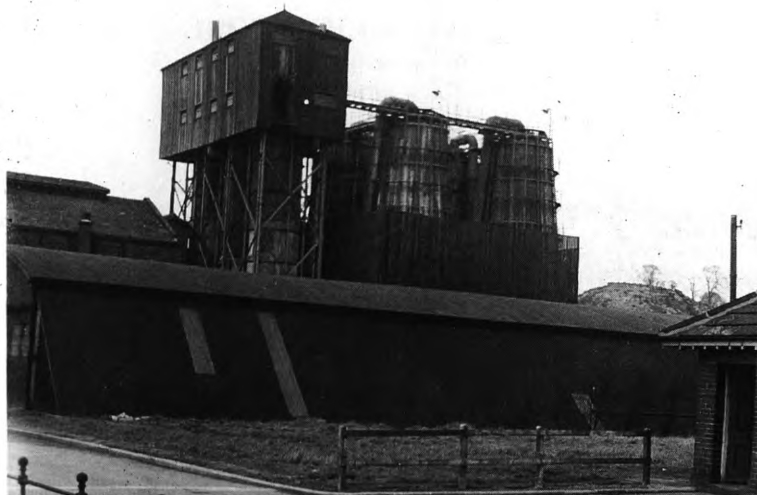
Figure 4. Lead chamber plant for sulphuric acid at Bradford, 1956.
