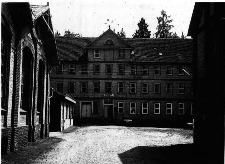
Figure 4. Osterode: Front of the main building of Greve & Uhl's woollen mill (Eulenburg), former carding and spinning floors, 1832; since c.1970 out of operation and temporarily used as office or storage facilities.
