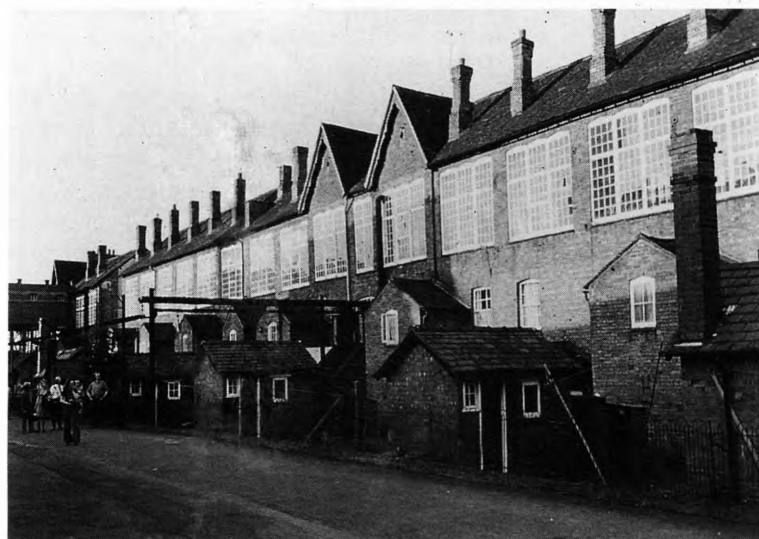
Figure 2. A row of 'cottage factories' constructed for the Cash Brothers in Coventry in 1857: the large windows imply the use of Jacquard looms. Power was supplied to the upstairs workshops from a central steam engine, whilst living accommodation was on the lower two floors.
