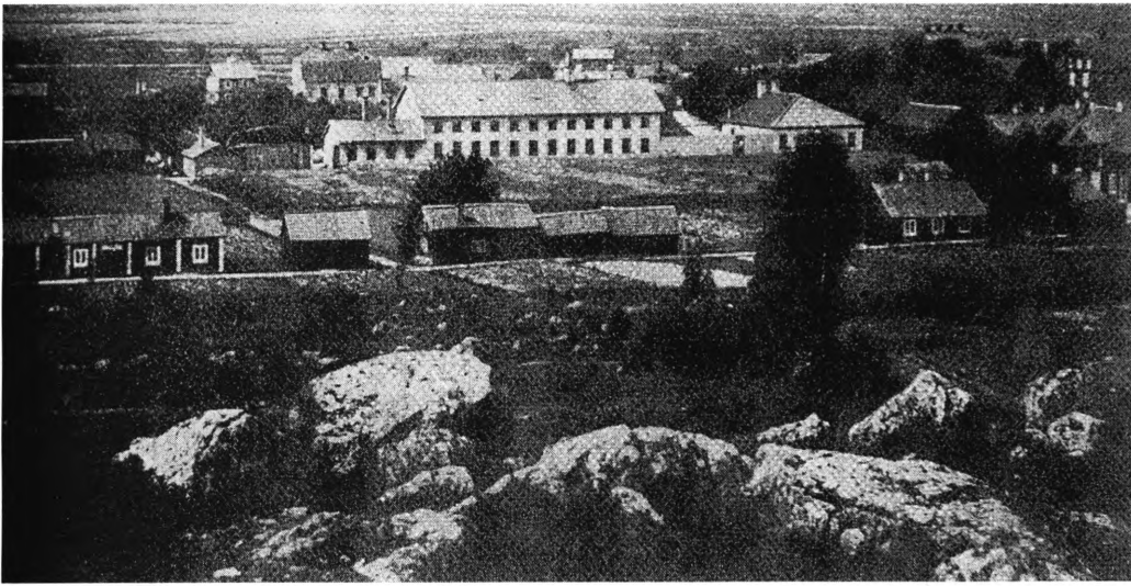
Figure 4. Köpings mekaniska verkstad in the 1860s. The machine shop, distinctly different from the surrounding buildings, is the large white building in the centre while the smaller one to the right was the foundry. Further to the right is the manager's house which was more modest than the owners' homes in Överum and at Ludvigsberg. Photo: Köpings mekaniska verkstad's archive, Volvo, Köping.
