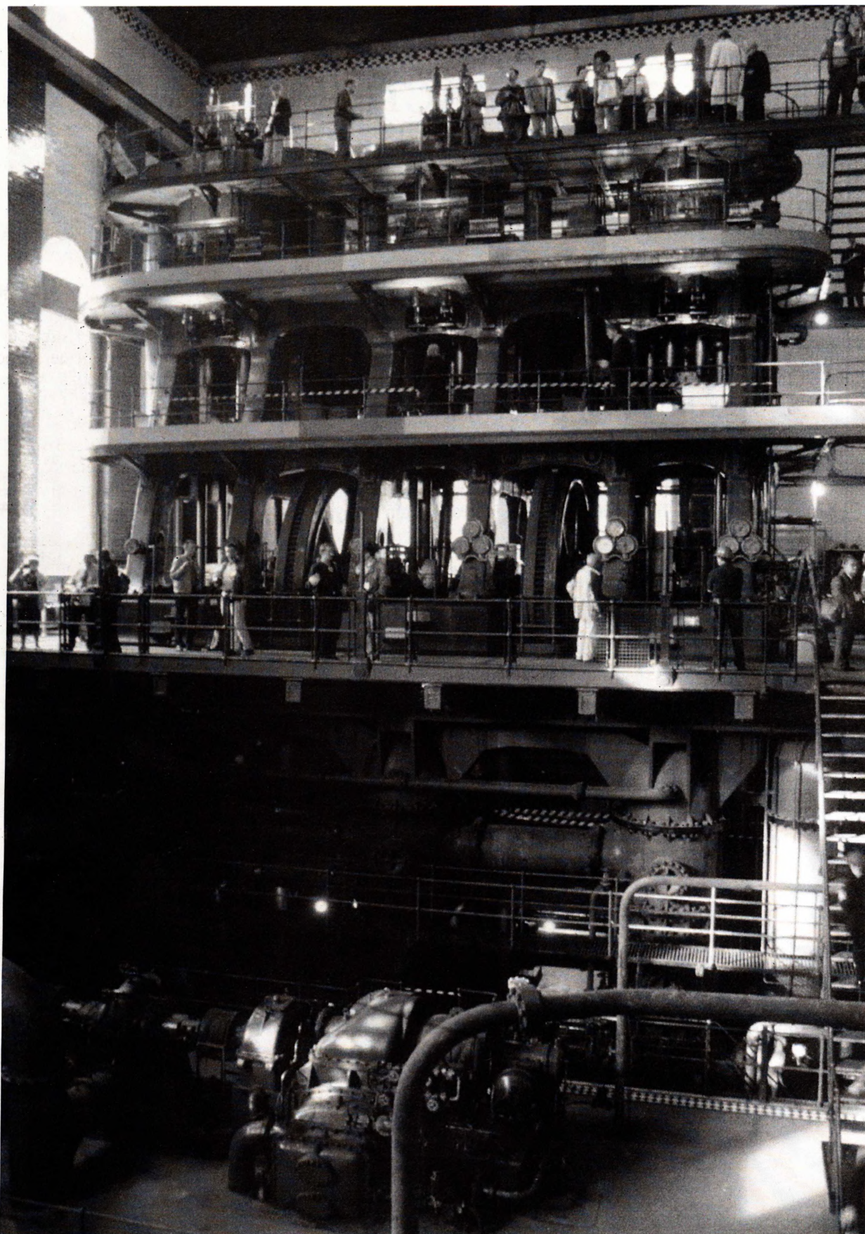
TICCIH2000 Congress delegates aboard one of the two triple expansion steam engines at the Kempton Park Pumping Station of the former Metropolitan Water Board. They were built by Worthington Simpson of Newark (Nottinghamshire), commissioned in 1928 and were in use until 1980. The Kempton Great Engines Trust was formed in 1996 and has now nearly completed the restoration of one engine to working order (Photo: Marilyn Palmer).
