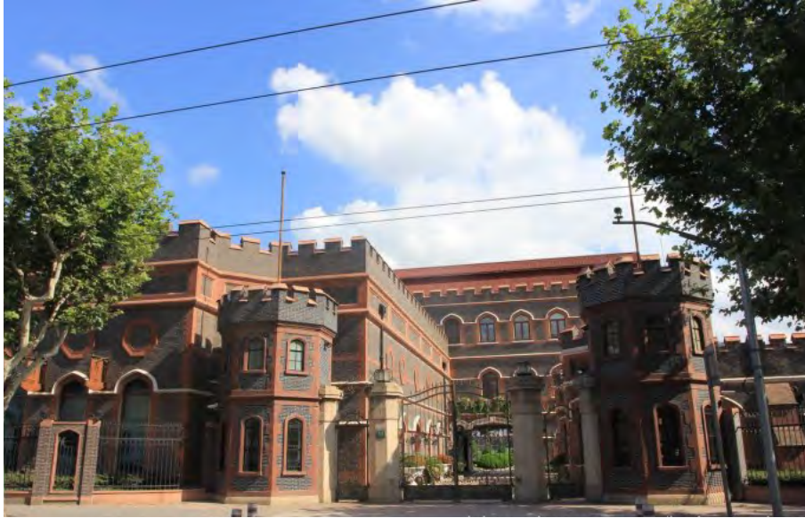
Shanghai Yangshupu Water Plant
