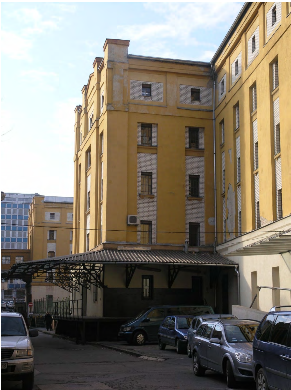
The impressive reinforced concrete warehouse building of the former Lágymányos tobacco factory, rehabilitated in Budapest. © Györgyi Németh, 2015
