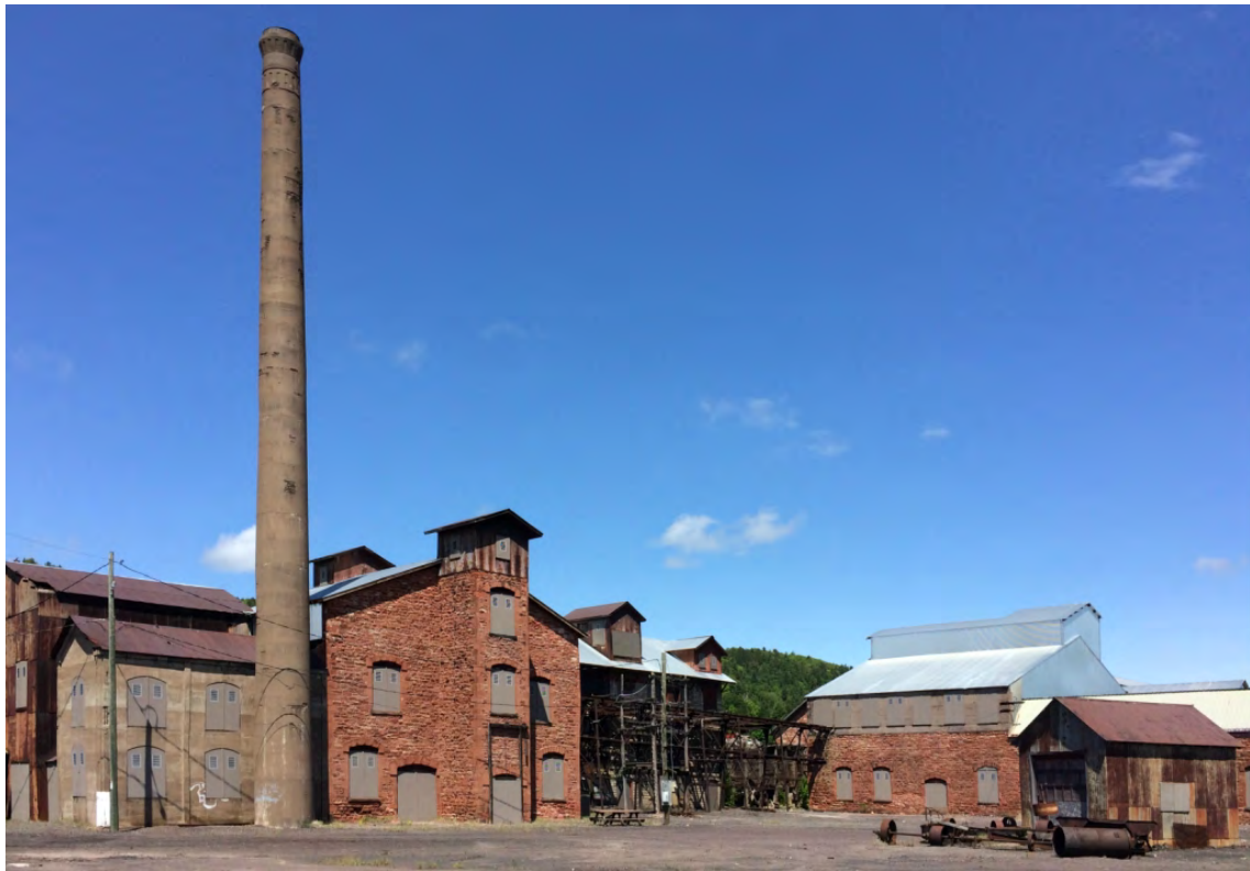
Quincy Smelter, part of the Quincy Mine National Historic Landmark, and soon to be incorporated into the Keweenaw National Historical Park that interprets copper and copper mining. © Scott See, 2015
