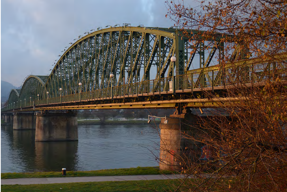
Combined rail/road-bridge across the Danube in the city of Linz.
