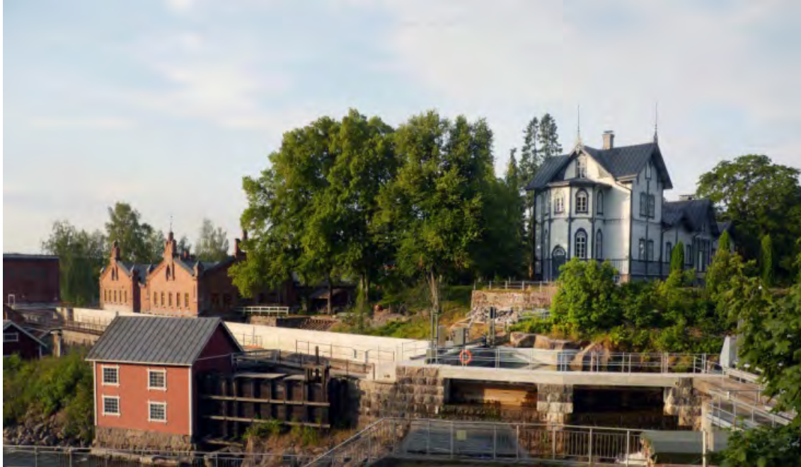
Verla rapids and the new shelter dam in the foreground. Verla groundwood and board mill behind. © Lassi Kujala 2014
