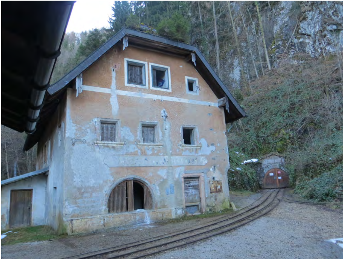
Wolfdietrich-Berghaus in Hallein before demolition.
