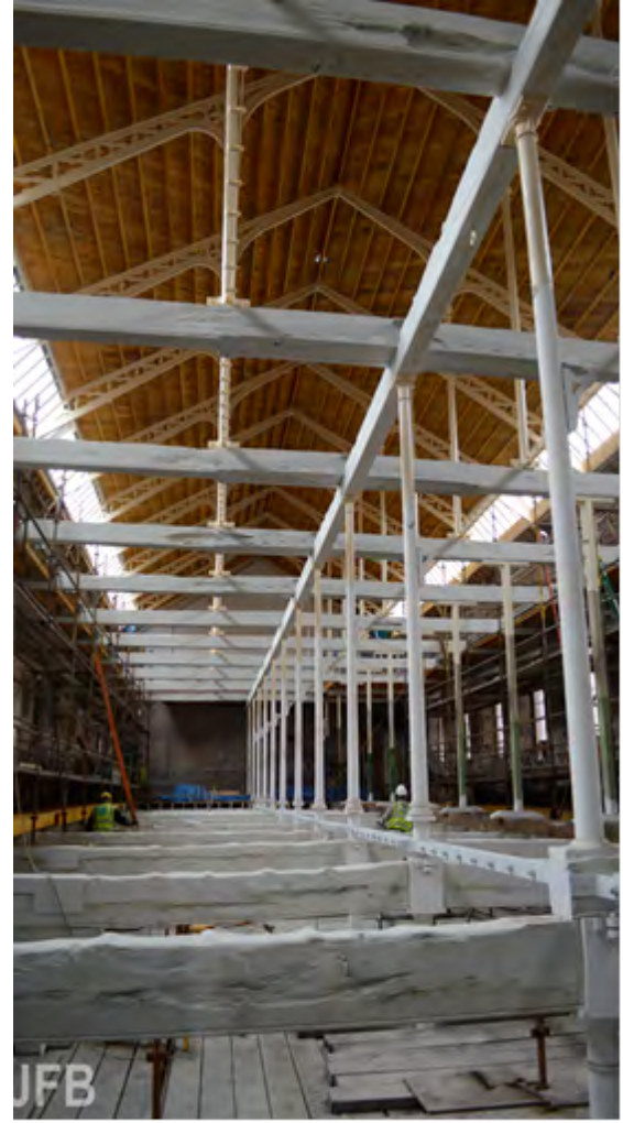
Verdant Works, showing the impression on the beams made by the now removed floorboards. 1833 with a Gothic cast iron roof of 1852. © Dundee Heritage, by Jim Burns.
