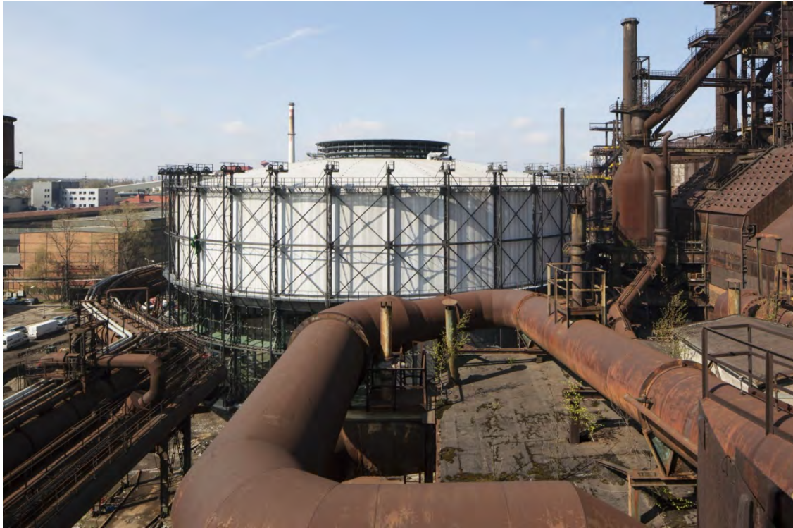
View of the gasometer at Vítkovice Ironworks in Ostrava, converted to Gong Multifunctional Centre in 2012. © Tomáš Souček
