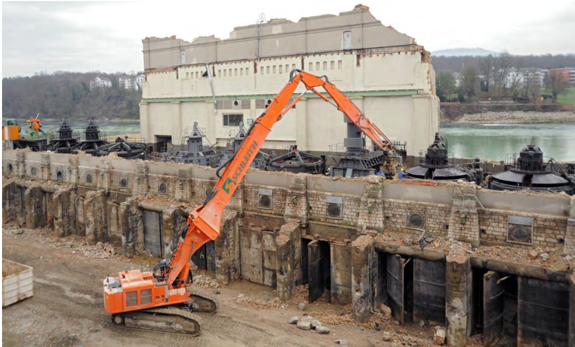
Demolition of the Rheinfelden Hydropower Station, 2011. © C. Bedeschinski
