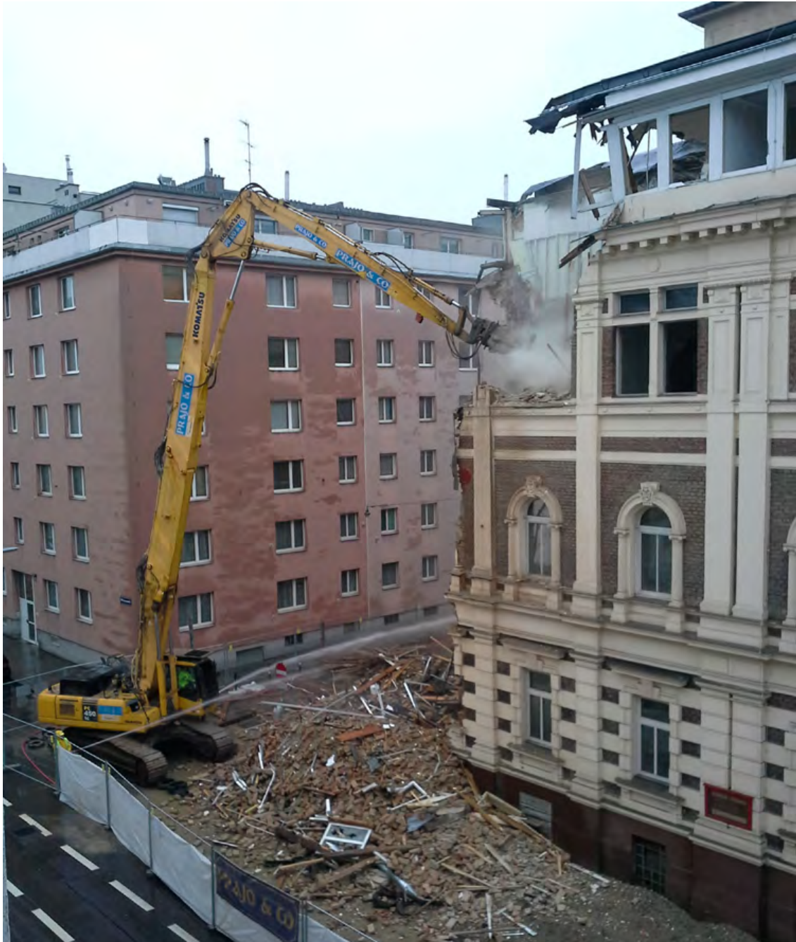
Demolition of former office building of Brown-Boveri-company in Vienna.
