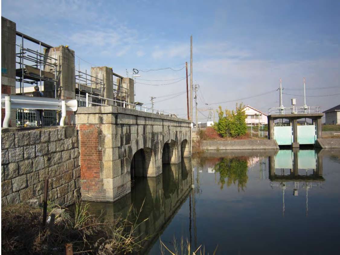
The triple floodgate of Hinoe-gawa (the river Hinoe was constructed in 1904. The Kojima-Bay reclaimed land make up to 11000ha from 1720's (in the middle of the Edo era) to 1963, (when reclamation works finished). © A. OITA / 16. Oct. 2014
