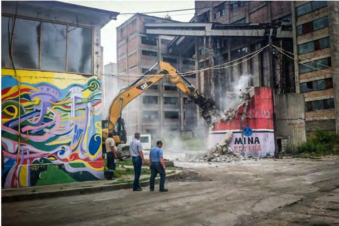
Petrila Mine the Jiu Valley in process of being demolished.
