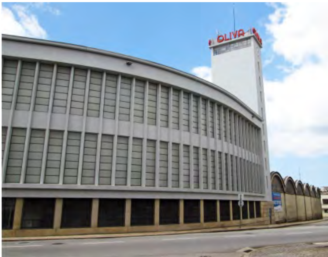
“OLIVA Tower” of the metallurgical factory OLIVA, now the Welcome Center of the “Industrial Heritage Routes at São João da Madeira”. © Carolina Castañeda López, 2014
