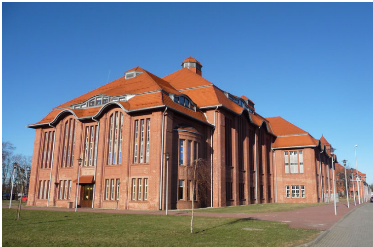
The Gliwice Coal Mine (Gleiwitzer Grube) miners' changing and engine halls resemble palaces rather than industrial buildings. Huge historical windows have been replaced with new ones and the original divisions preserved
