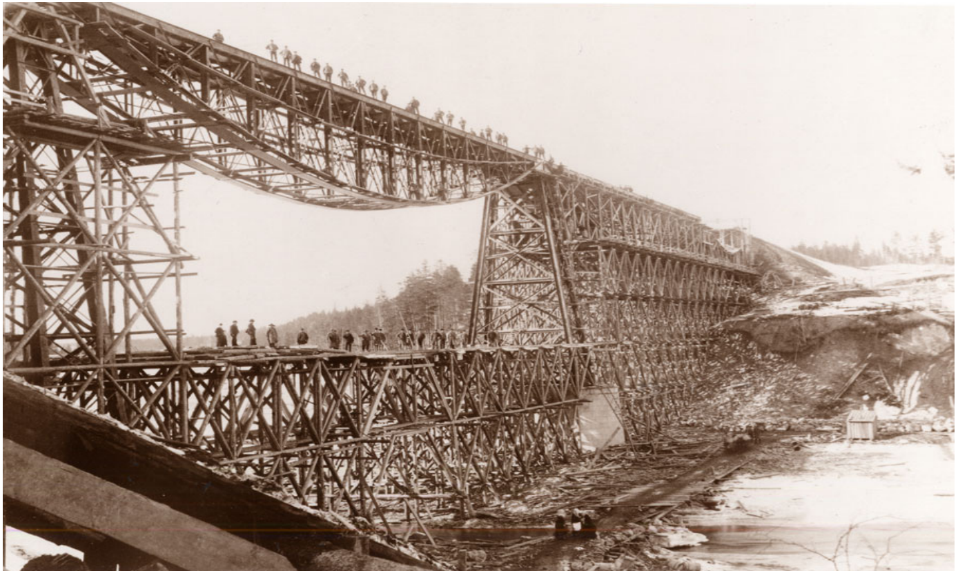
Construction of the railway bridge over the Vindel river in 1892.
