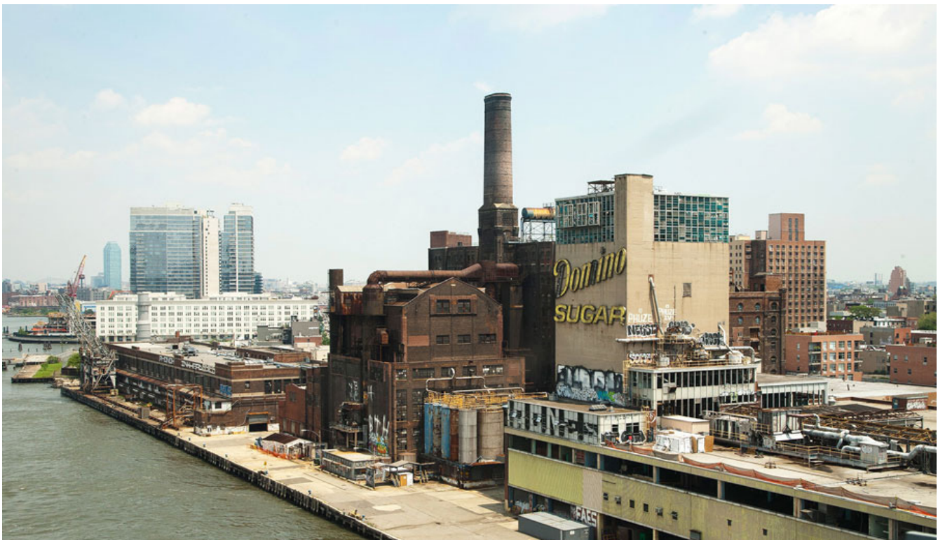
The Domino Sugar Factory from the Williamsburg Bridge prior to demolition in October 2014.
