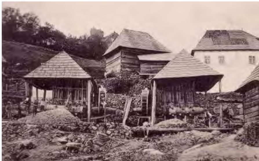
Traditional stamping mills; at the communist nationalization, in 1948, more than 400 such installations existed; they were all destroyed
