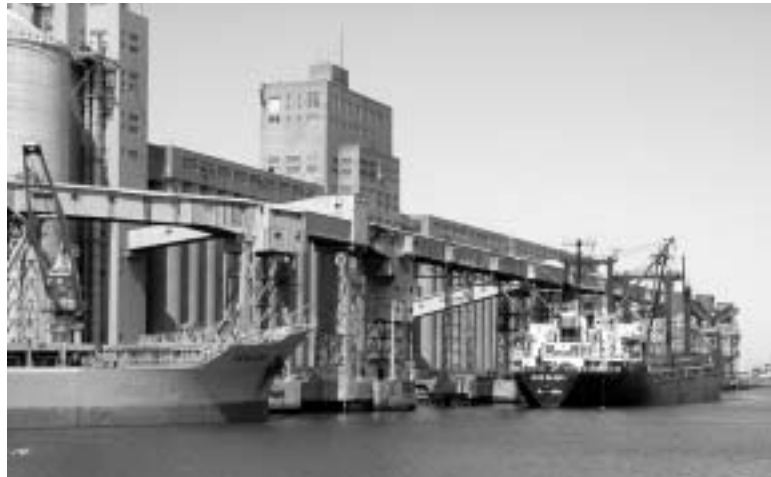
Silos and warehouses in the port area of Necochea-Quequén, Buenos Aires
