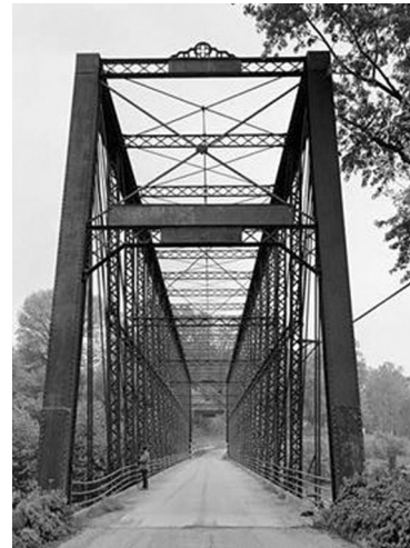
Laughery Creek Bridge (1878), Aurora, Dearborn & Ohio Counties, Indiana, was fabricated by the Wrought Iron bridge Company of Canton, Ohio, another of the prolific metal truss bridge fabricating companies that competed in the fierce iron bridge market during the last quarter of the 19th century. With a construction depth of 40ft, Laughery Creek Bridge has an exceptionally long span of 300ft for a simply supported parallel chord truss. The bridge is the only triple-intersection Pratt surviving in the US. HAER Collection, Library of Congress.
