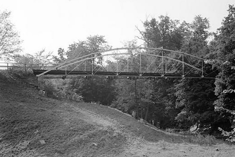
Whipple Cast & Wrought Iron Bowstring Truss Bridge (1867), Normanskill, Albany County, New York, was patented by Squire Whipple in 1841 and was one of the first scientifically designed iron bridges in America. The photograph illustrates the quintessence of Whipple's revolutionary design - every member was mathematically sized to handle its respective load, resulting in an extremely light, material-efficient, gravity-defying structure. HAER Collection. Library of Congress. See Eric Delony's Report .
