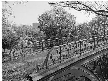
Gothic Arch (1864), New York, New York. While the Civil War raged in the South, English architect Calvert Vaux and English engineer Jacob Wrey Mould were assisting American landscape architect, Frederick Law Olmsted, in completing construction of Central Park in New York, which included a collection of cast-iron arches separating equestrian from pedestrian traffic. Five of these elegant bridges survive, representing America's best collection of decorative cast-iron arches. While this type of bridge was common in Europe, especially England, they were an anomaly in the United States. American bridges were usually of parallel-chord truss construction made up of standard structural parts — angles, channels, plates, and eye bars held together by rivets and pins to facilitate shipping and assembly at the site. HAER Collection, Library of Congress.
