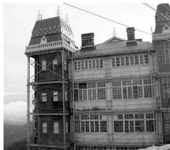
The Railway Board in Shimla, the summer capital of the British in India was made entirely of cast iron from England and designed by engineers who worked on the Crystal Palace in London.
