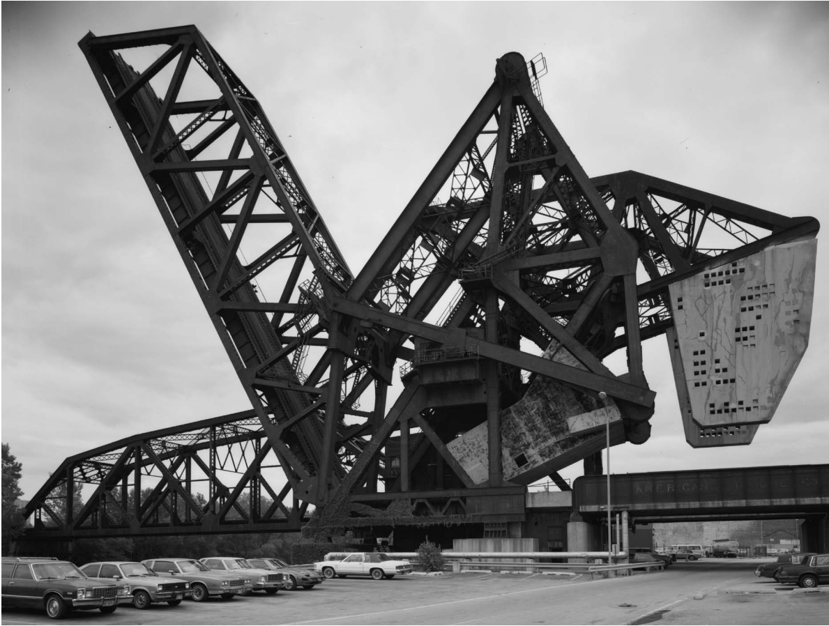
The Baltimore & Ohio Railroad's bascule bridge over the Chicago River at the Chicago Terminal is one of many engineering and industrial landmarks in the city. Photo Credit: Historic American Engineering Record
