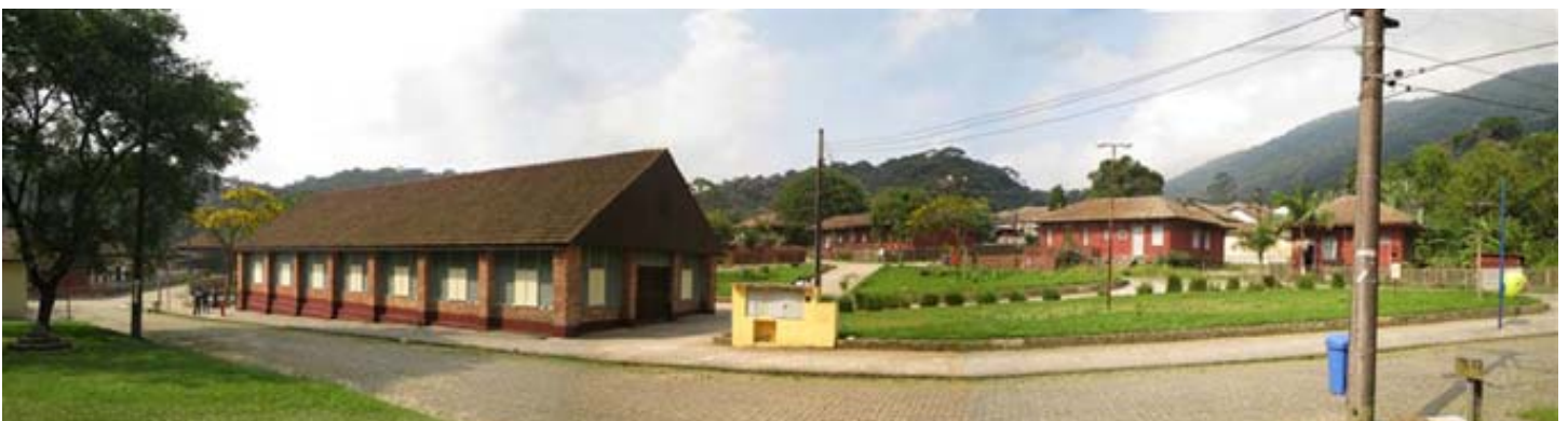
The houses were built with setback front gardens, something uncommon in Brazil at this time.
