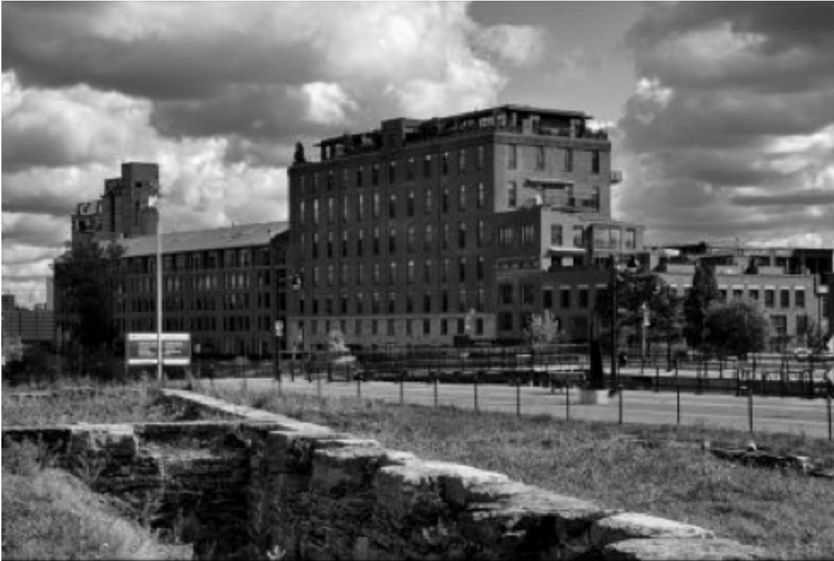
The former Dominion Textile Mill in Saint-Henri, Montreal, has also been converted into condominiums. Photo credit: David W. Lewis.
