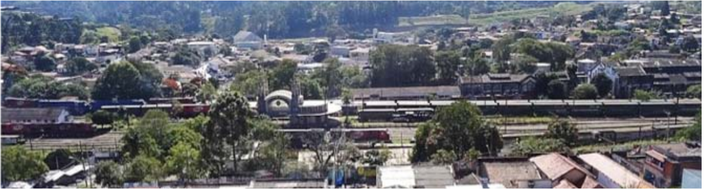
Panoramic view of Mairinque village railway station, with the station in the center; workshop buildings on the right and the railway village in the foreground. Photo: Rafaela Rondon Rogato Silva, 2017.
