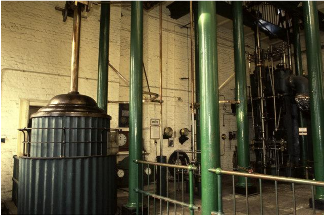
The 1820 Boulton & Watt beam engine, one of two originally installed at Chelsea Pumping Station beside the river Thames in London and moved upstream to the Kew Bridge pumping station in 1840. Photo: Chris Allen, Creative Commons
