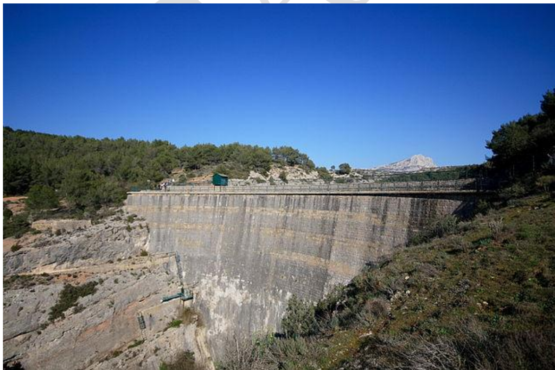
The Barrage Zola is an early masonry arch dam built to supply Aix-en-Provence following a cholera epidemic in the city. Creative Commons
