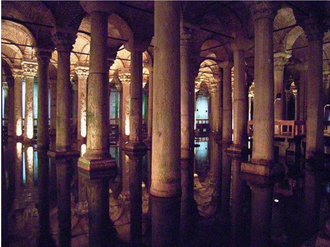
Recycled columns support the vaults of the Yerebatan cistern in Istanbul. Water was brought 19 km through channels incorporating two Roman aqueducts. Robert Raderschatt, Creative Commons
