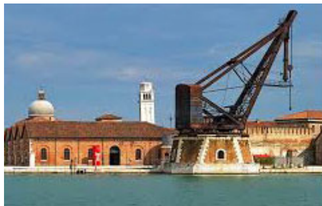
The Armstrong hydraulic crane in the Venice Arsenale was designed in 1893 to help service the ironclad warships of the Italian navy. The rivetted steel structure, rollers, rails and rotation platform, is suffering severe corrosion and needs urgent conservation treatment - see Report on industrial rust
