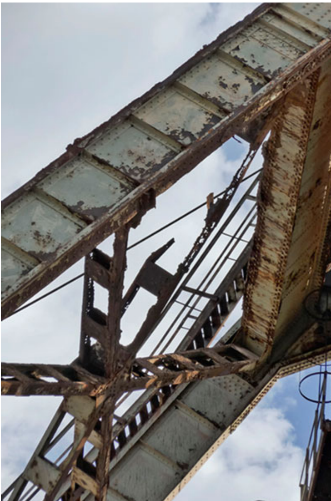
Friedrich-Wilhelm shaft head frame. Surface and erosive corrosion grade B-D in the cross brace. Initial damage was by an operational accident in 1994
