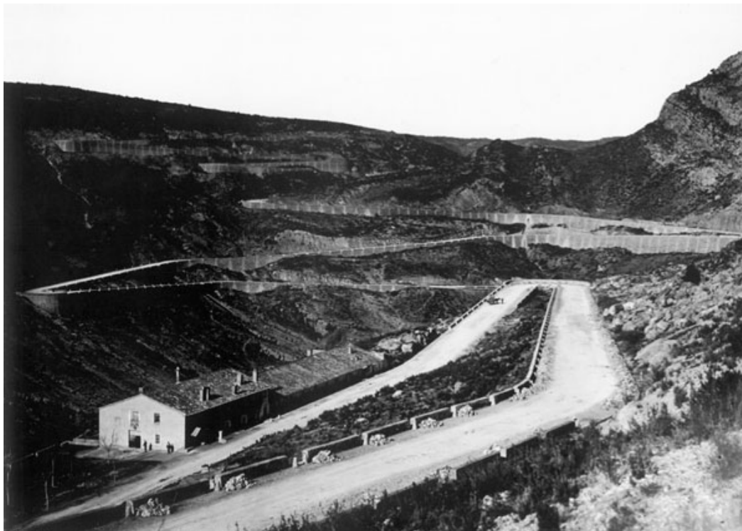
The Contreras mountain pass between Madrid and Valencia, Spain. This section was designed and built by the engineer Lucio del Valle in the mid-19th century. Its aim was to provide access, as far as possible, to a point on the Mediterranean coasts to allow the supply of goods from Valencia and Catalonia to Madrid in the most effective and economic manner.
