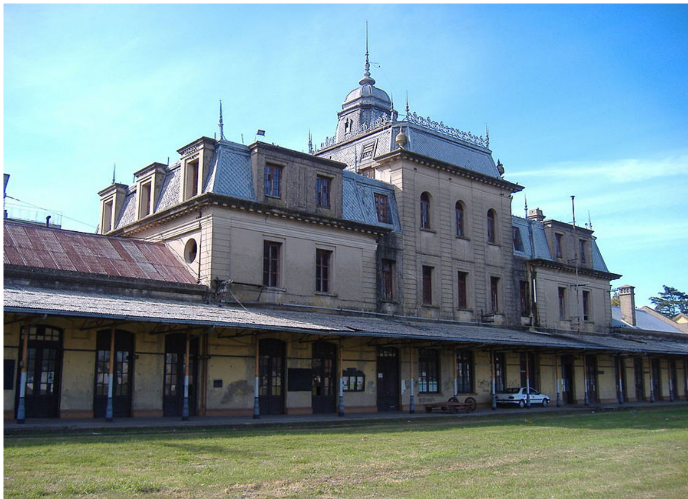
Rosario central station dates from 1888 and was partly rebuilt in 1921. The centre of an urban park since 2005, the new national rail company plans to spend A$ 15m restoring the building. Photo: Pablo D. Flores, Creative Commons
