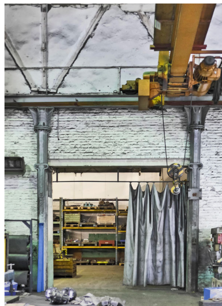
The interior of the oldest conserved part of the foundry was probably built around 1850. The lower parts of the columns are made of then-already standardized iron supports, while the upper section is a timber frame construction.
