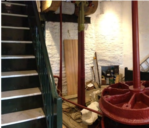
Elsecar pumping engine near Barnsley, the piston ready to go back into the cylinder. © Industrial Heritage Consulting Ltd
