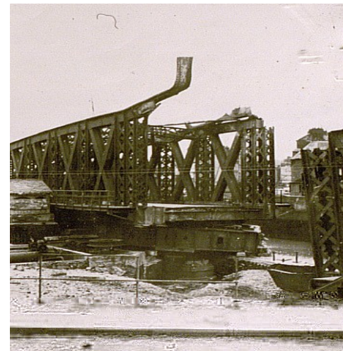
The Colbert bridge on September 1944 The main structure was destroyed on a 12 meters length, the mechanism has partly suffered. After the quay being strengthened by Allies, the bridge reconstruction begun. It took nearly two years to achievement because of the shortage of raw materials after the war. Below, rare photos showing the bridge rebuilding site. Note that the original operating instruments stayed intact.
