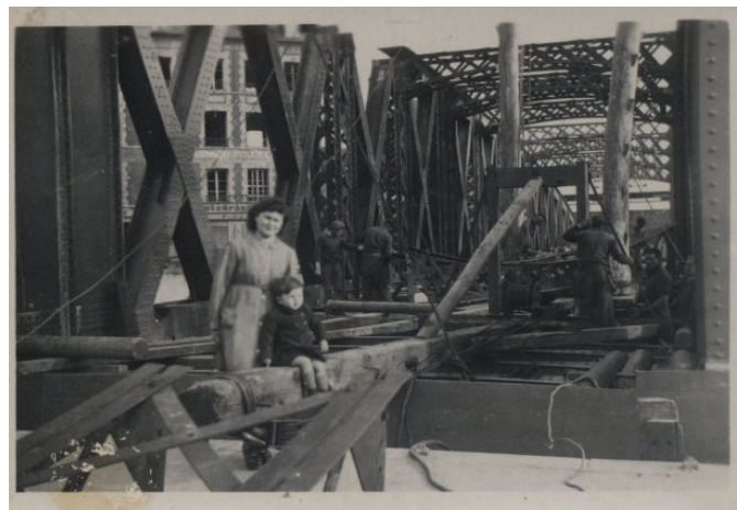
The Colbert bridge on September 1944 The main structure was destroyed on a 12 meters length, the mechanism has partly suffered. After the quay being strengthened by Allies, the bridge reconstruction begun. It took nearly two years to achievement because of the shortage of raw materials after the war. Below, rare photos showing the bridge rebuilding site. Note that the original operating instruments stayed intact.
