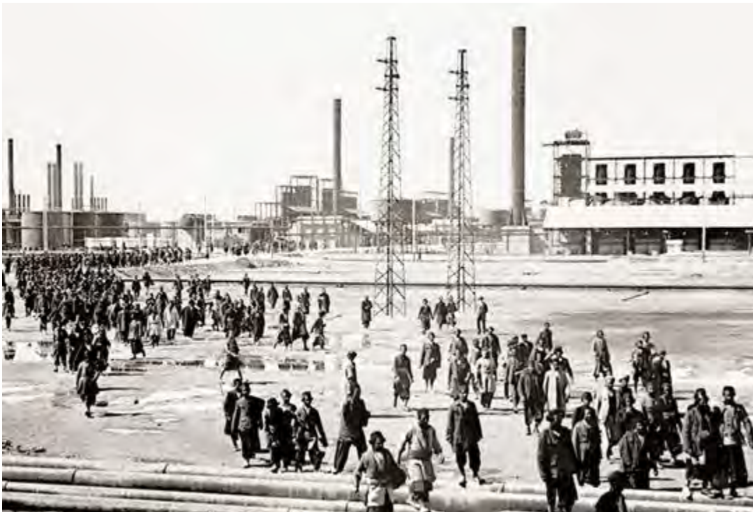
Abadan Oil Refinery
