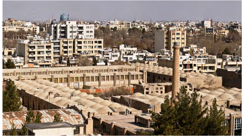
Risbaf textile factory, surrounded by new construction Isfahan, Iran
