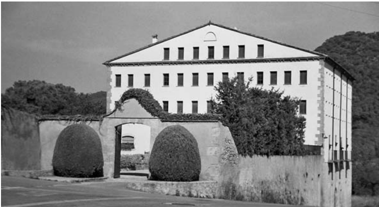
The Munné paper mill in Capellades, the last of a dozen 18th and early 19th century mills closely spaced along a small rec or power canal. The very typical typology of the mill has drying spaces on the upper two floors, accommodation for the family in the middle while the production of pulp and sheets of paper took place in the basement.
