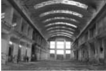
The Torroja factory near Madrid, an early reinforced concrete shell vault by the Spanish engineer Eduard Torroja on the Spanish threatened sites list.
