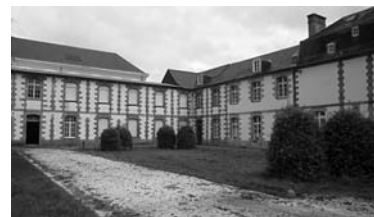
Up. The remarkable snuff grinding mills.
