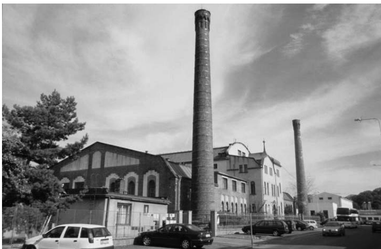
Bubeneč sewage works, Prague, now an eco-technical museum. Paul Smith
