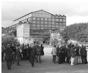
The Lavoir de Chavannes coal washing plant. (Photo Denis Varloot)
