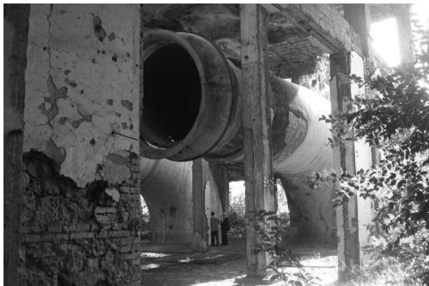
Actual view of the horizontal wind galleries.
