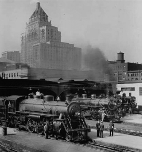
Toronto Union Station, Canada, c.1930. East end of train shed with Royal York Hotel in background. Source: Archives of Ontario
