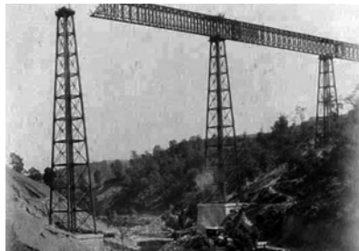
Malleco Viaduct: construction of the structure in 1889
