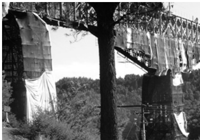
Restoration of the viaduct during 2006
