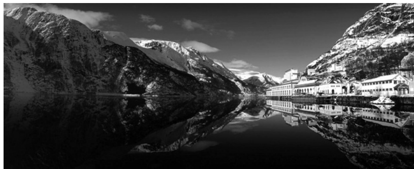
Tyssedal power plant on the Hardangerfjord, Norway
