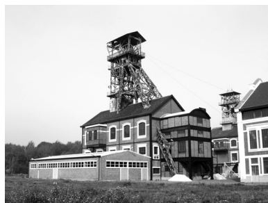
The former Oignies Colliery (9-9), proposed for partial adaptive re-use as a truck-stop. Photo: Dr Stephen Hughes
