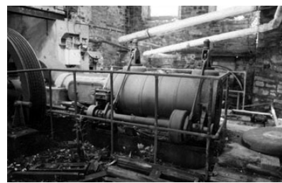
One of two Robey Uniflow steam engines installed during the tannery phase, and still on the site.
