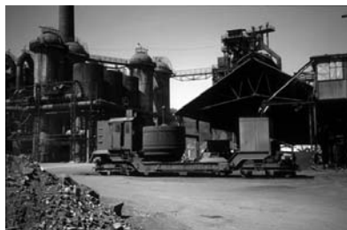
The Maxhuet plant in Sulzbach-Rosenberg, Bavaria, Germany
