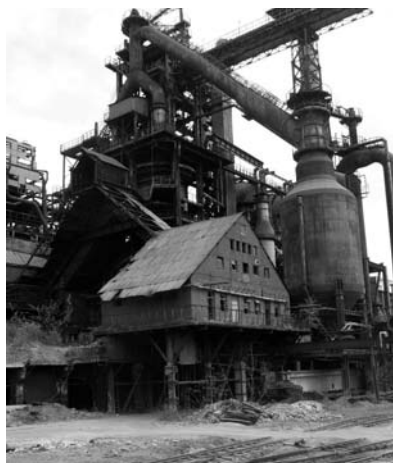
TKM Resita blast furnace, founded in 1962. Photo: Mark Watson.
