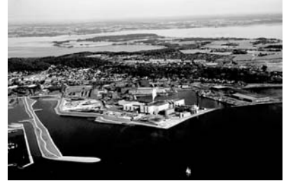
To document of large technical system like this steel works in Denmark is a job for specialists. The built-up area is on more than 143.000 m 2
