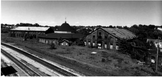
1998 view of the Martinsburg Shop complex before work began.
